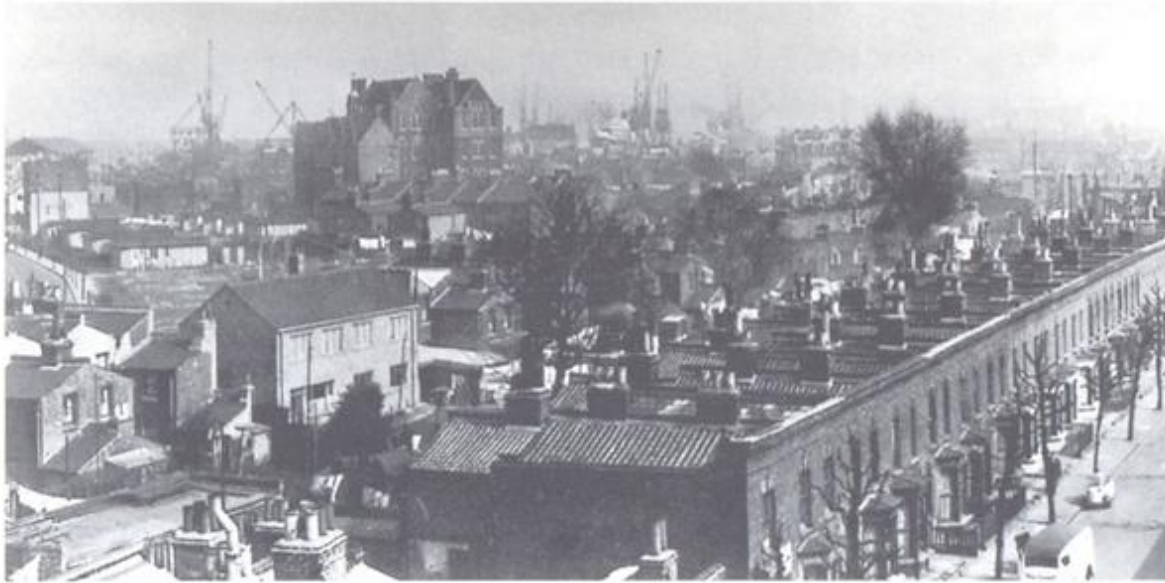
Figure 4.1: Board school in South London, seen in situ
