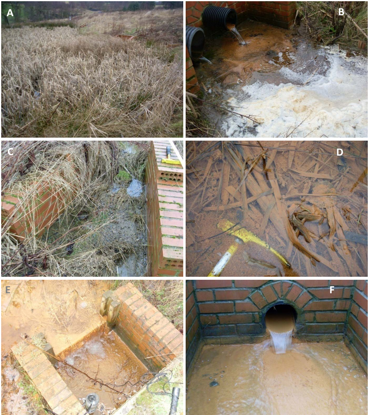
Figure 4 The wetland is overgrown by Typha latifolia and Juncus effusus (A) and receives mine water from overflows and effluents of the RAPS (B). In addition, agricultural runoff is collected in a channel surrounding the treatment site and in seasons of high precipitation discharges additional water into the wetland (C). The wetland (D) and the outlet chamber of the wetland (E) are covered by reddish precipitates. Some staining was also observed at the final discharge point into Willington Burn (F).
