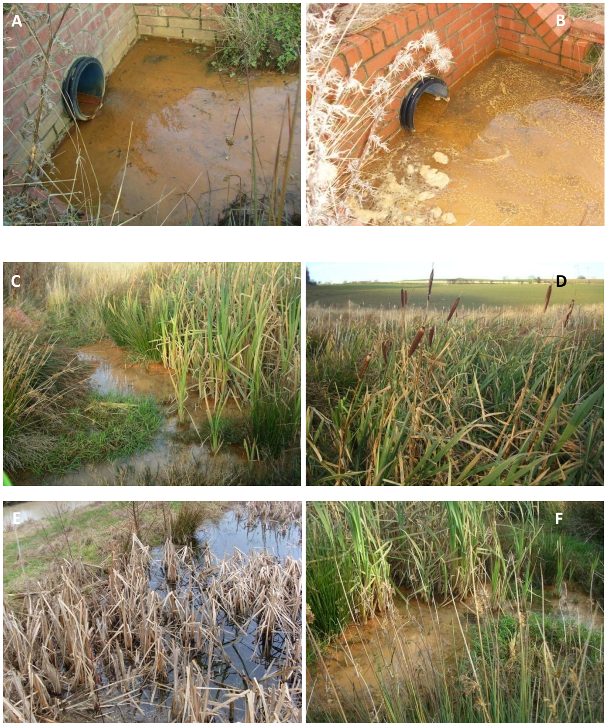
Figure 1 Images, taken in October 2007 and January 2008, show the Reducing and Alkalinity Producing System 1 (RAPS 1) with seasonally dependent inflow rates (A, B). The water is characterized by high turbidity and reddish colour. The water is backed up around the influent chamber rather than distributed equally throughout the RAPS. Typha and other wetland species have established on the system through natural succession and contribute to the accumulation of organic matter (C-F).
