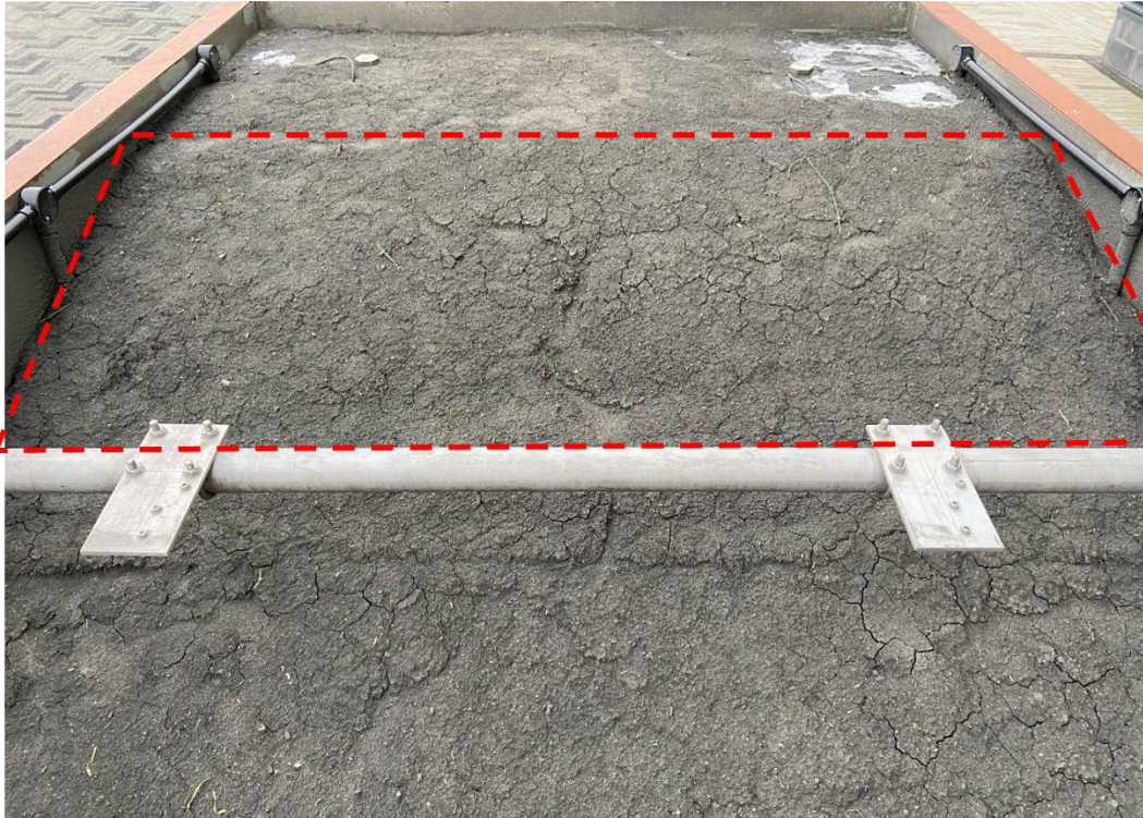
Figure 4.8: Photograph illustrating the emergence of desiccation cracks on the central upper region of the lysimeter slope (red box) due to its prominence relative to surrounding slope regions and minimal interference from the physical bounds of the lysimeter container.
