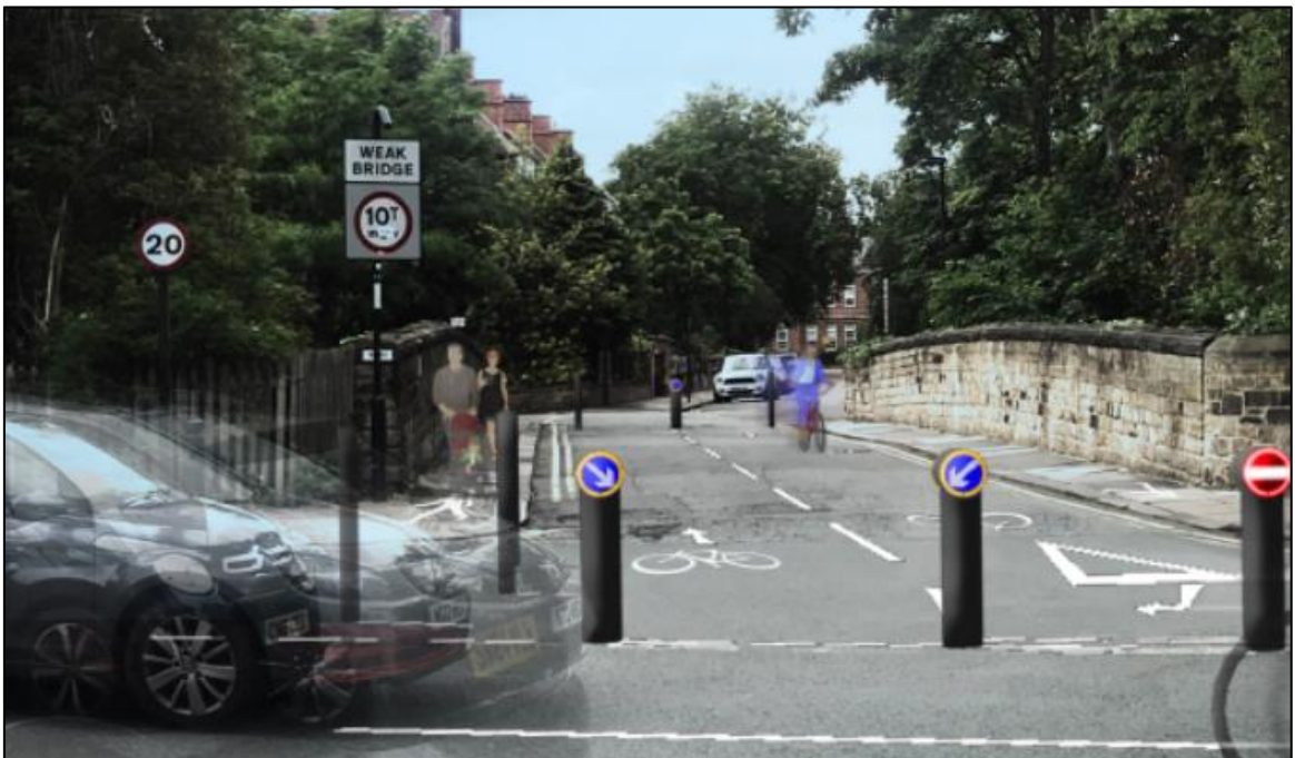
Figure 6.5 Haldane Bridge after Measures (Newcastle City Council, 2021).
