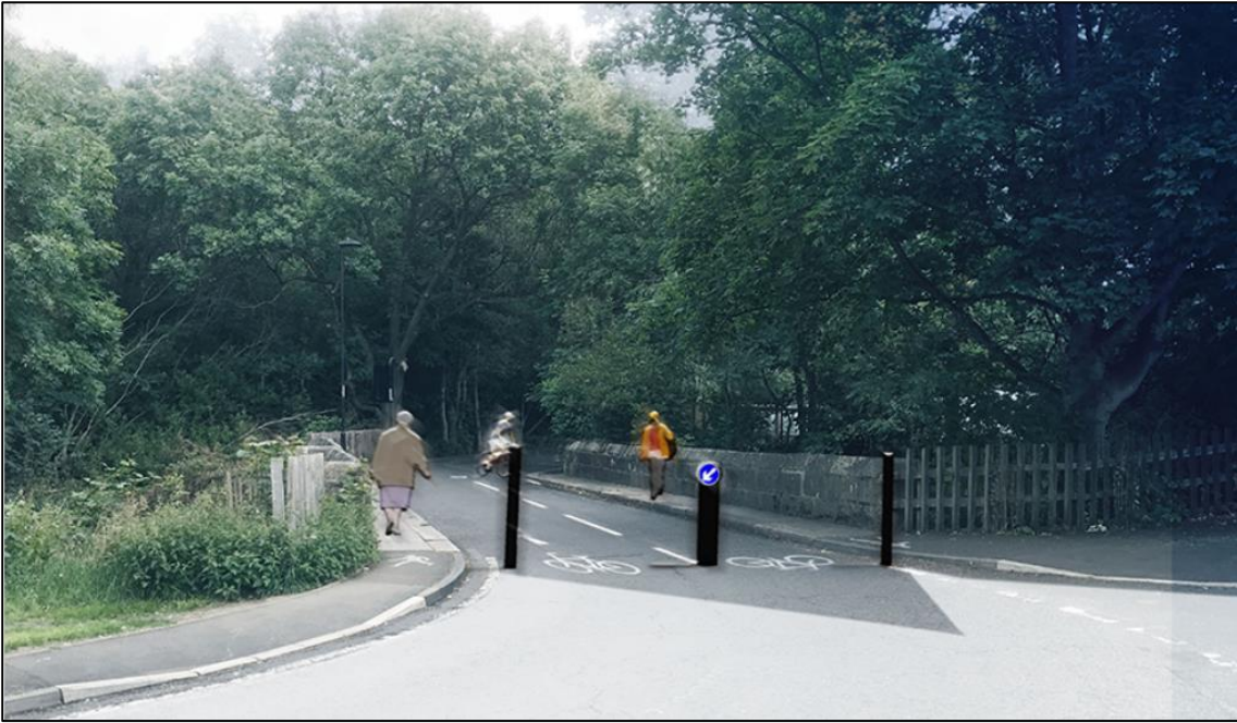
Figure 6.11 Salters Bridge after Traffic Calming Measures (Newcastle City Council, 2021).
