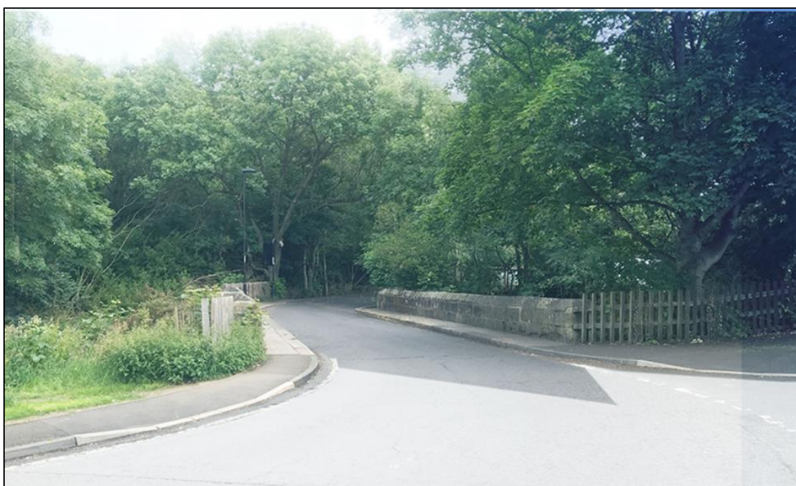
Figure 6.10 Salters Bridge before Traffic Calming Measures (Newcastle City Council, 2021).
