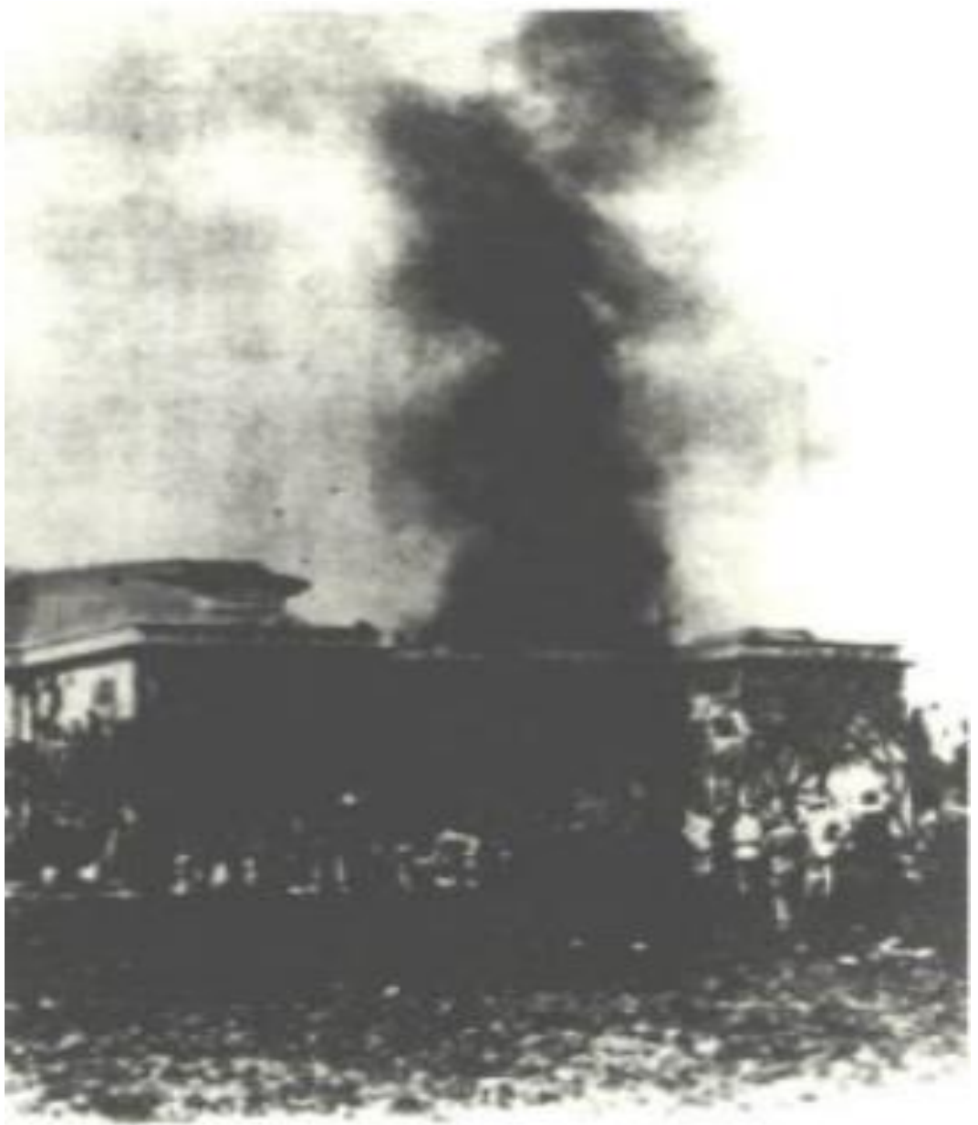
Plate 6.1 The library building of the Hunan University. Source: Tian Fulong 田伏隆, ed., Hunan lishi tudian san 湖南歷史圖典三 [Hunan historical atlas, volume 3] (Changsha: Hunan meishu chubanshe, 2012), 289.
