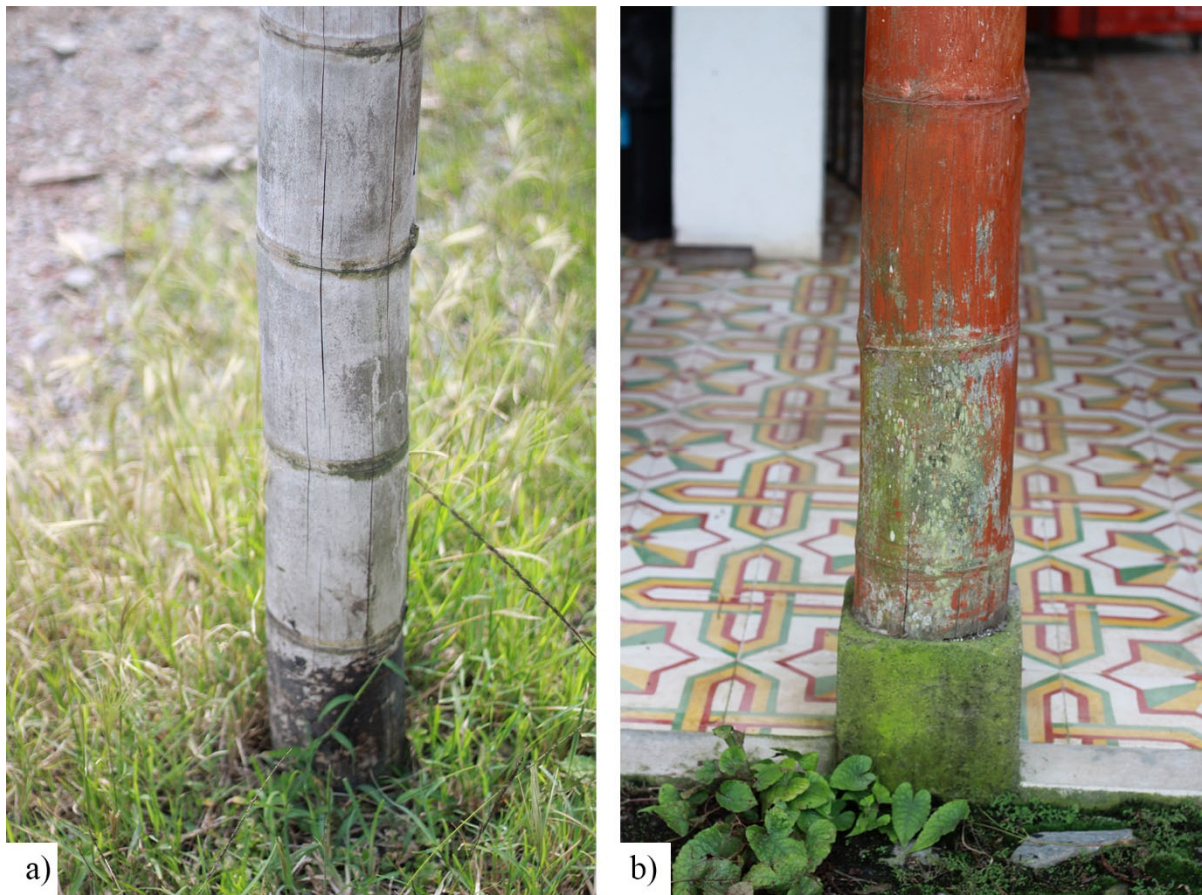
Figure 38: (a) Bamboo pole placed into the ground, and (b) the effect of rain splashing at the lower portion of a bamboo column even though it is raised above the ground. Photos by author, 2022.
