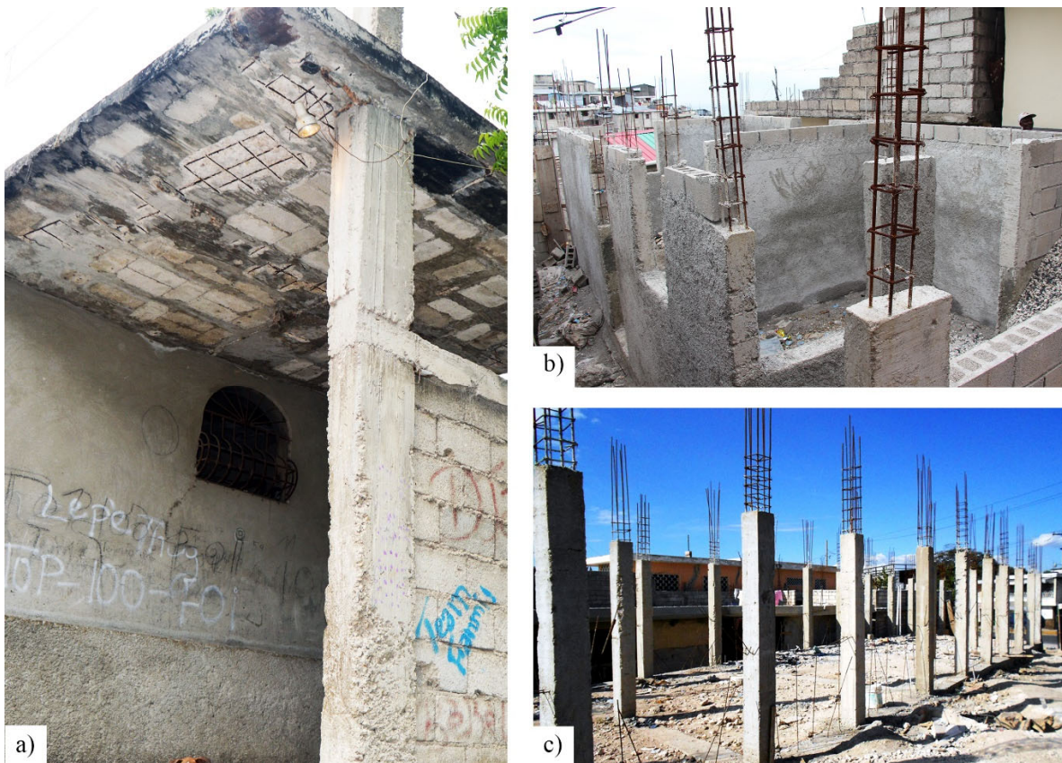
Figure 17: Images of construction taking place in Port au Prince, Haiti: (a-b) Construction with CMUs in Baillergeau, Port au Prince, Haiti, and (c) reinforced concrete columns under construction, Delmas, Port au Prince. Photo taken in 2012 and 2016 by the author.
