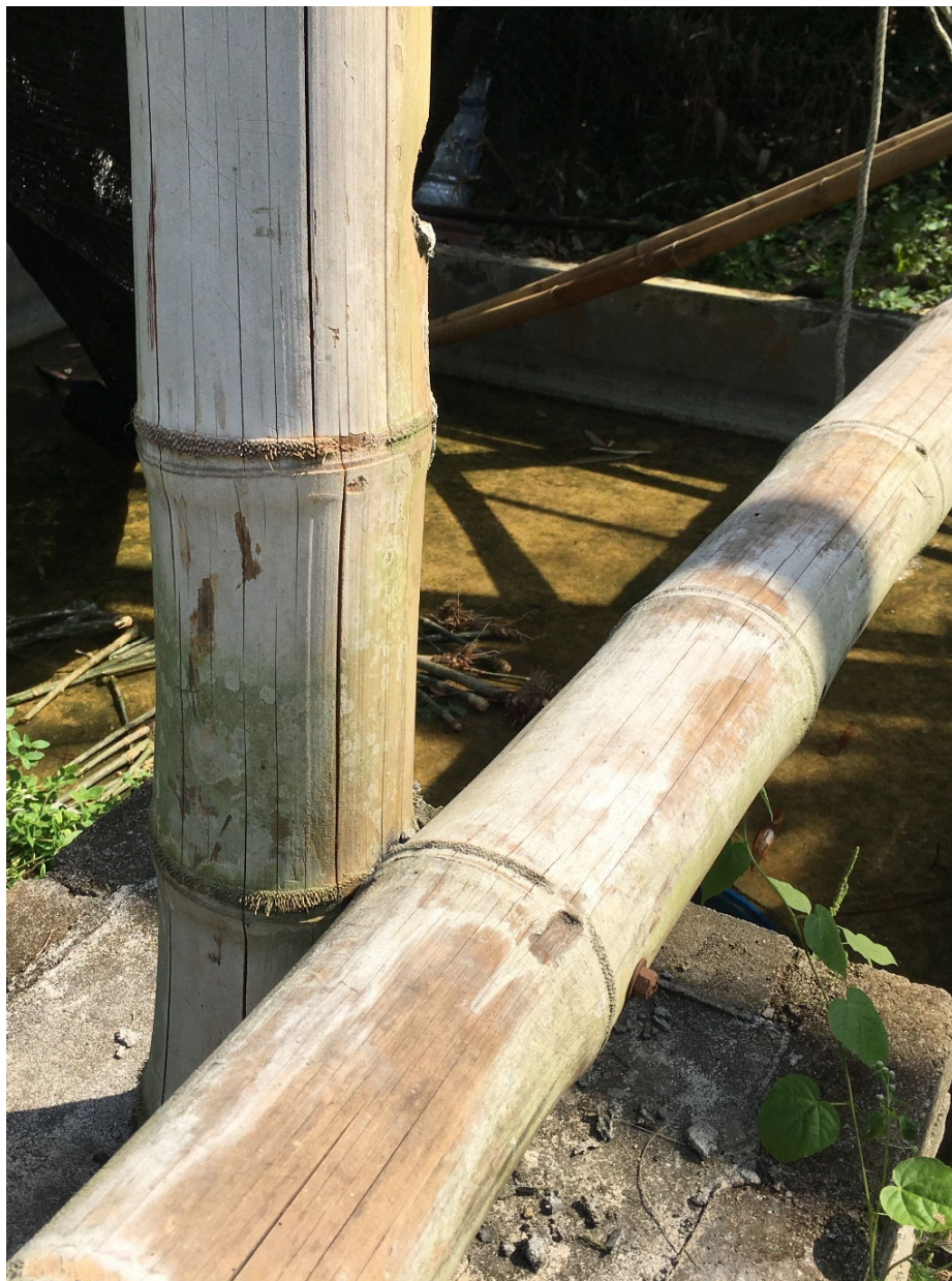
Figure 35: Bamboo poles exposed to UV light and rain, showing longitudinal splitting, or fissures. Photo by author, 2020.
