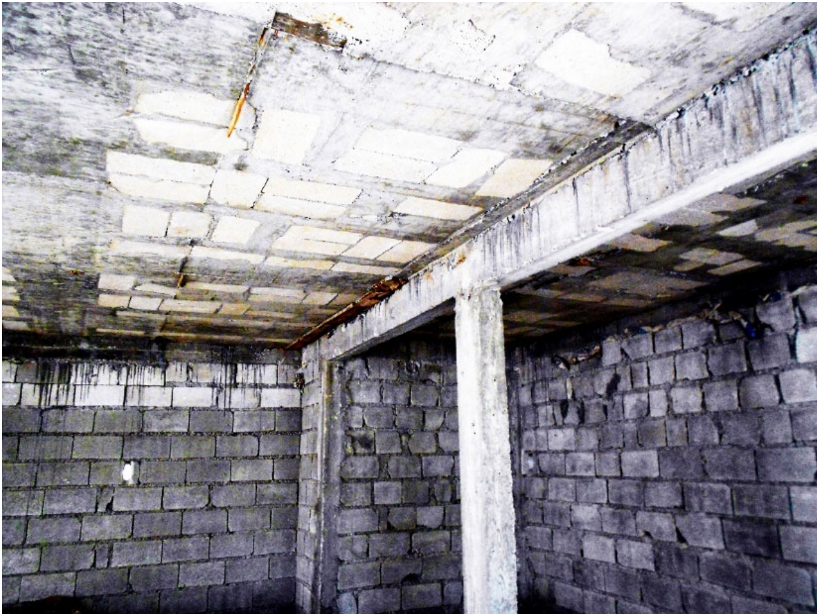
Figure 18: Chalky limestone aggregates used in construction in Port au Prince, Haiti, in 2012, two years after the devastating earthquake of 2010. Photograph by author, 2012.
