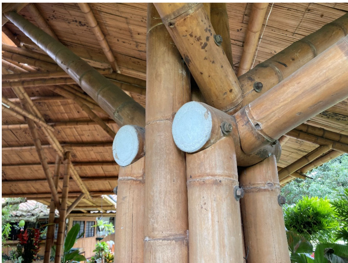
Figure 62: A mortar filled joint with the ends of the cut bamboo culm filled with mortar which prevents insects and moisture penetrating the bamboo culm. Photo by author, Ecobamboo bamboo treatment facility, outside Candelaria, Valle del Cauca, Colombia, 2022.
