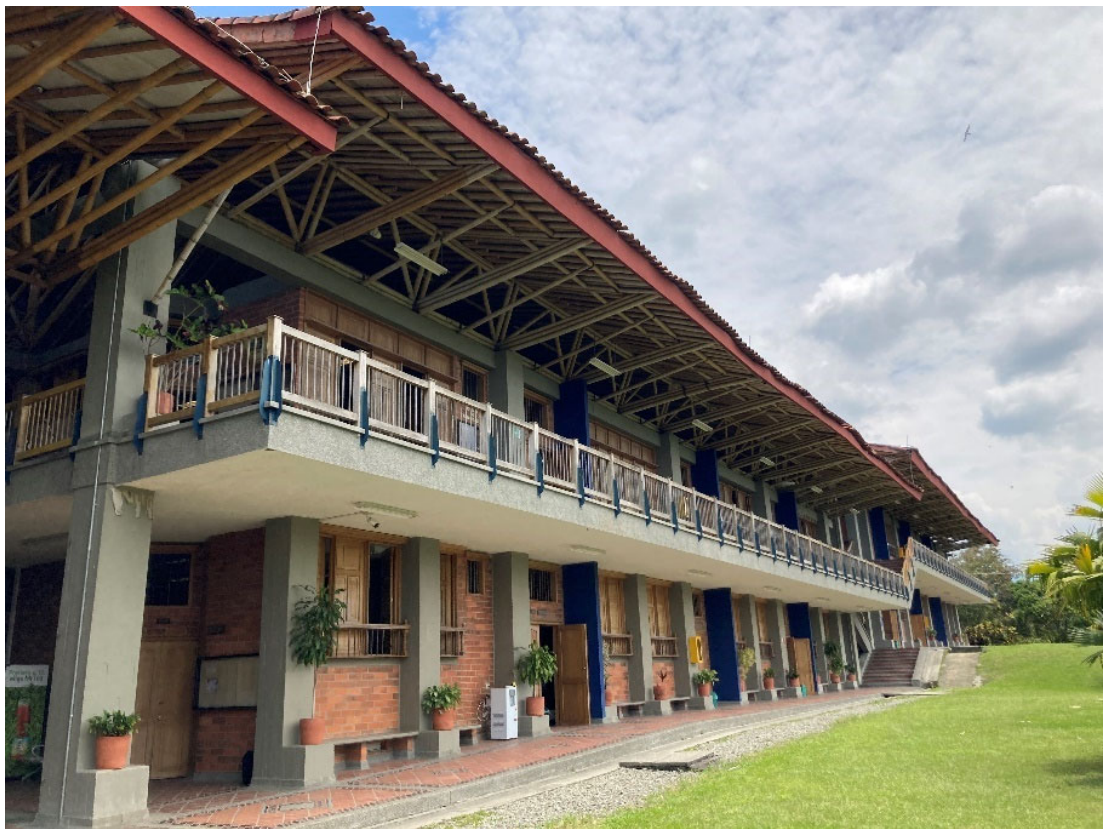
Figure 48: Roof overhang and masonry lower story, of the University of Gran Colombia, Armenia, Colombia. Photo by author, 2022.
