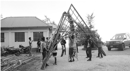
Figure 3: Construction of a small structure with locally sourced bamboo on the 2017 course.
