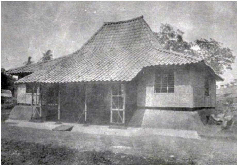
Figure 24: Model for a Javanese house executed with application of the purely wilah system for both the substructure and the roof grating. Caption and photo reproduced from Maclaine Pont (1922).
