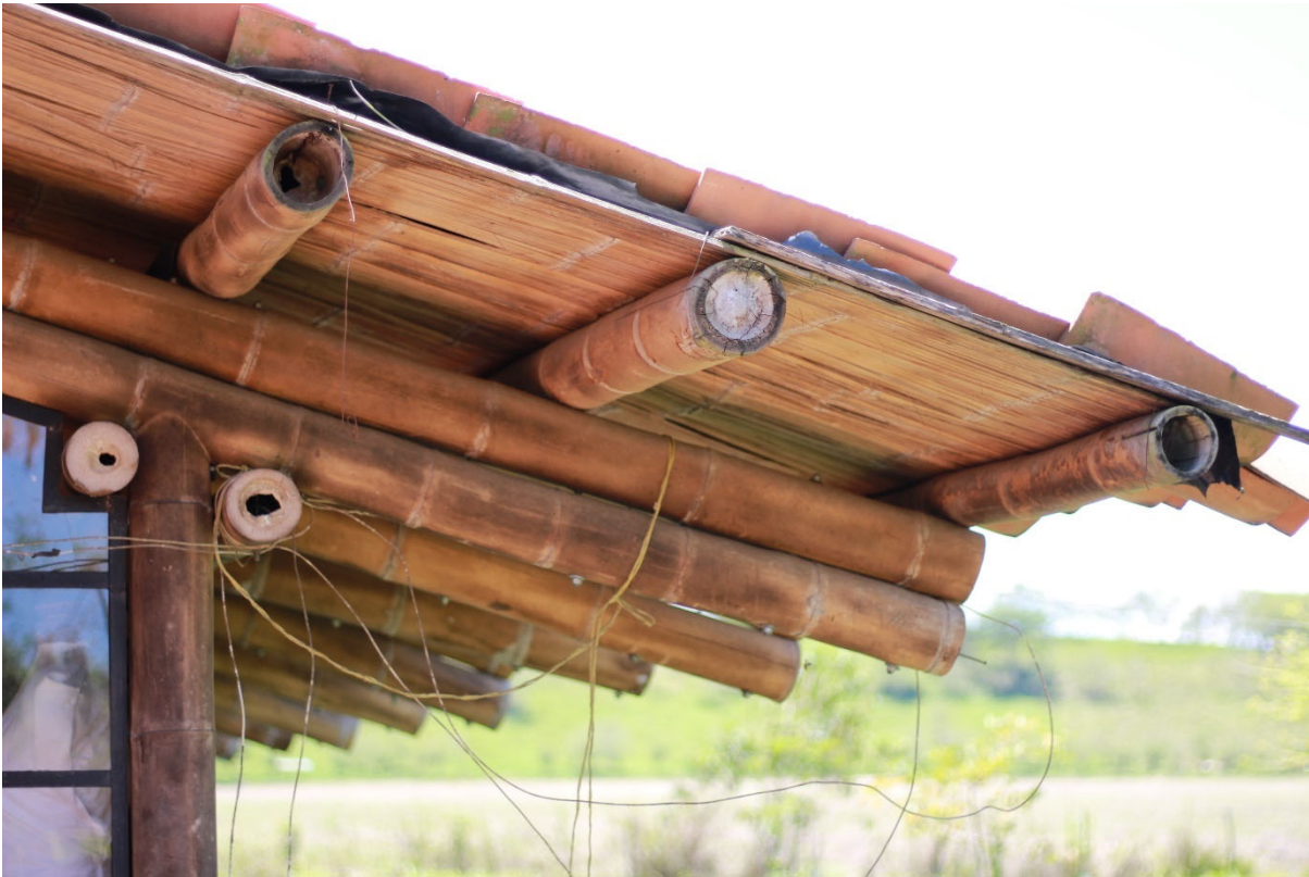
Figure 39: Bamboo purlins degraded at the edge of the roof eaves. Photo by author, 2022.
