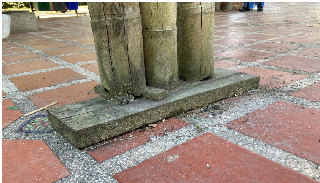
Figure 40: Bamboo poles in contact with a timber upstand on insufficient height. Photo by author, 2022.
