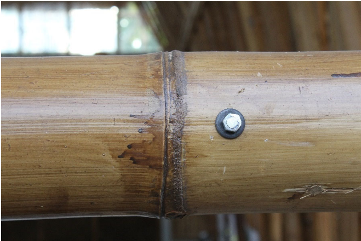
Figure 63: Bolting near to a node. Photo by author, 2019.
