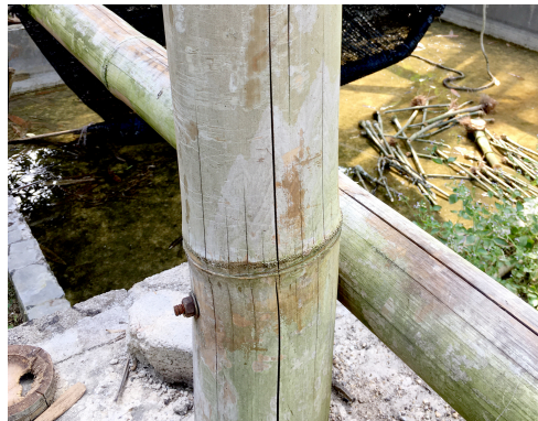
Figure 2 Full-culm bamboo poles cracked and showing signs of mould due to exposure of excess moisture and bleaching due to sunlight exposure. Photograph taken by author in 2020.
