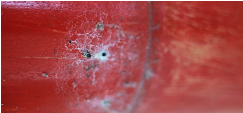
Figure 53: A painted bamboo structural member with a small hole covered in cobwebs where insects have burrowed. Photo by author, 2022.
