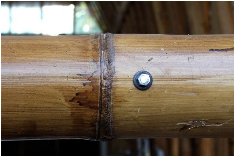
Figure 26: A bolt correctly located around 1 to 2 inches from the node.
