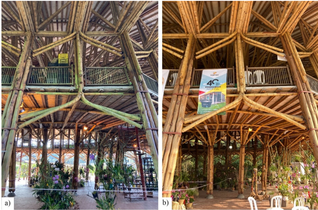
Figure 44: Comparison of two sections of the façade of the ZERI Pavilion : (a) showing a face of the façade facing the forest/vegetation, and (b) a face of the façade facing south, away from the forest. Photos by author, 2022.
