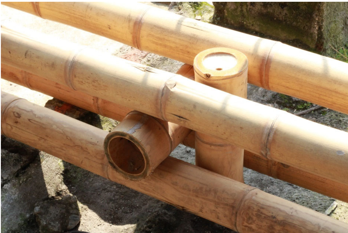
Figure 61: A four pole column, shown on the ground prior to erection. Photo by author, 2022.
