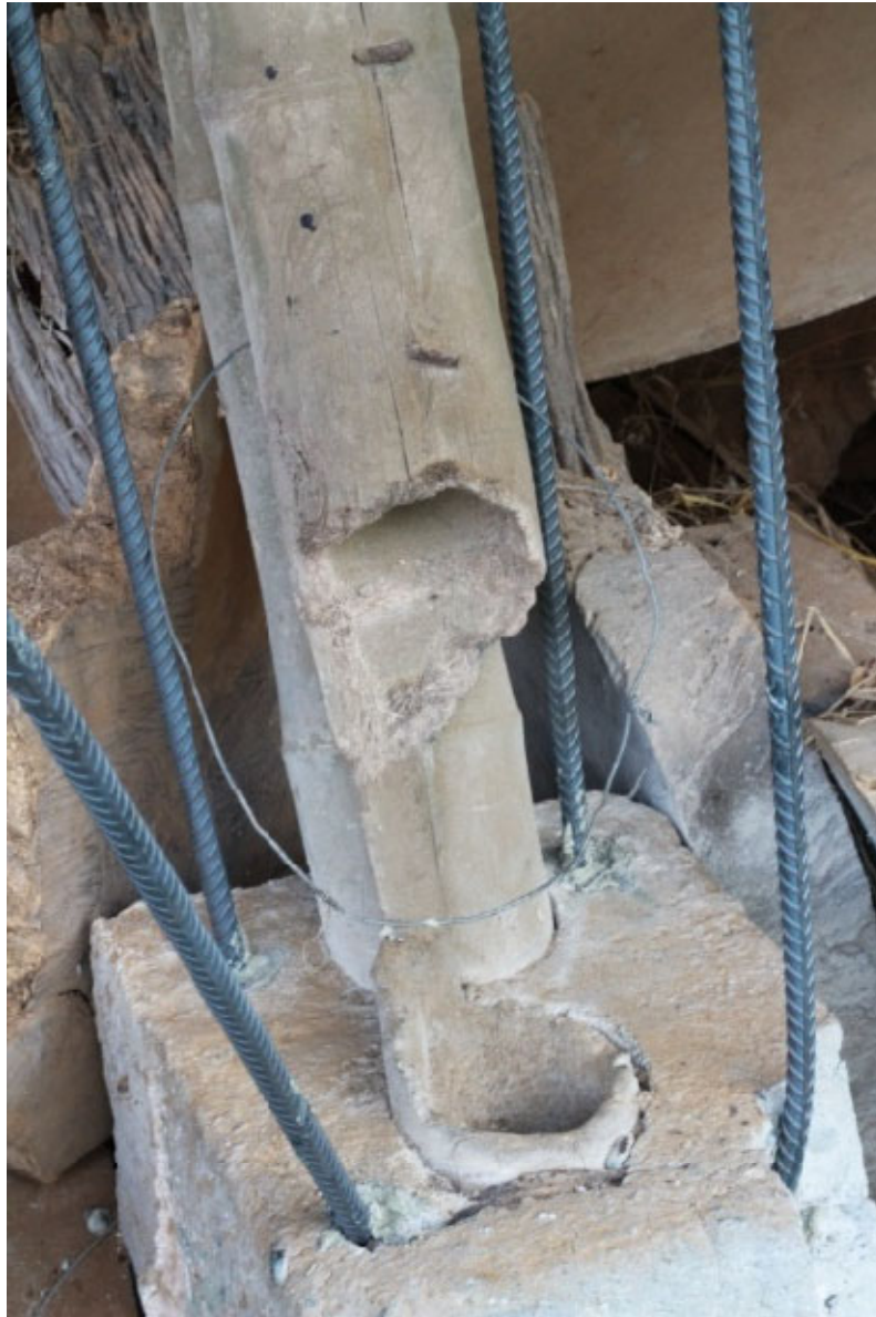
Figure 52: A bamboo column where the base has likely seen termite attack and the bamboo has been eaten away.
