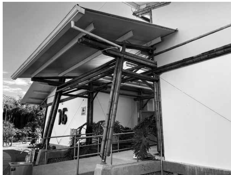
3 The bamboo species of Guadua angustifolia is well documented in the Colombia building code. Bamboo is the primary structural material in some campus buildings at the Universidad Tecnológica de Pereira, in Pereira, Colombia.
