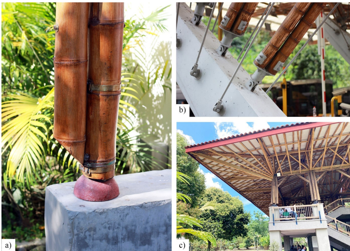
Figure 41: Good practice examples of raising the bamboo above the ground: (a) Concrete foundations at UTP, Pereira, Colombia, (b) piaje (tollgate) outside Manizales, Colombia, and (c) The University of Gran Colombia, Armenia, Colombia. Photos by author, 2022.
