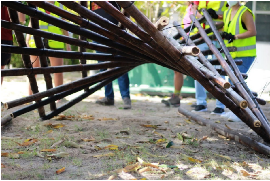
Figure 104: Image of hyperbolic paraboloid constructed during the Panama workshop in January 2022 from full-culm bamboo. Photo by author, 2022.
