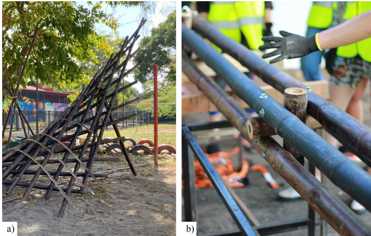
Figure 108: Physical one-to-one scale construction during the Panama workshop of two of the structural systems explored in the workshop: (a) hyperbolic paraboloid, and (b) four pole column to support a planar truss. Photos by author, 2022.
