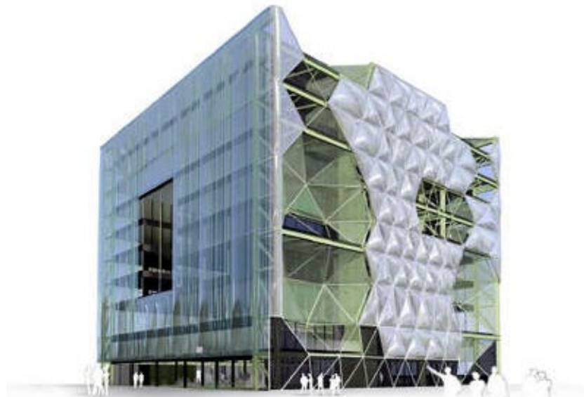
Figure 19: Media-Tic building and the use of pneumatics (EFTE) in large scale.
