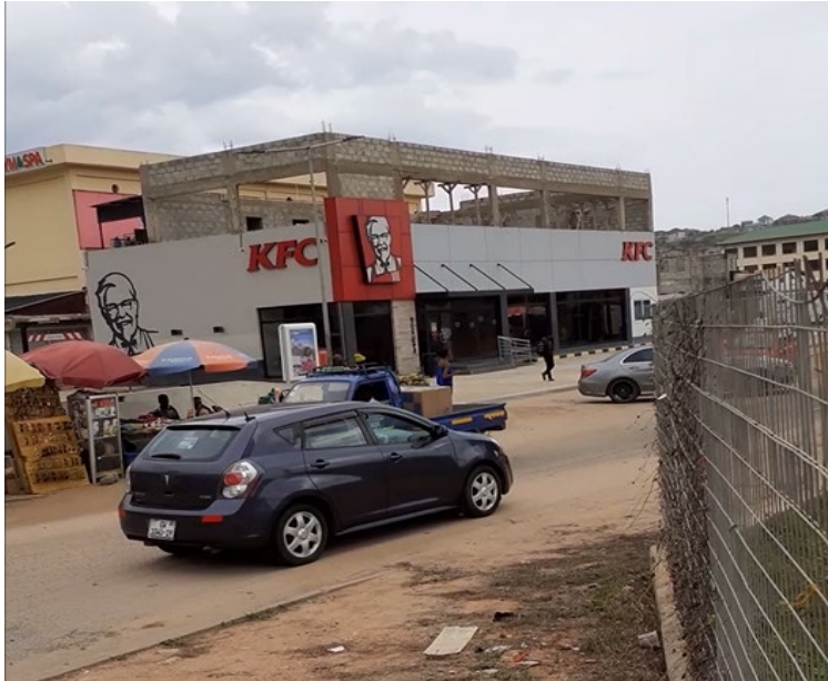
Figure 8. 9 KFC (Weija Branch) Undergoing Expansion.
