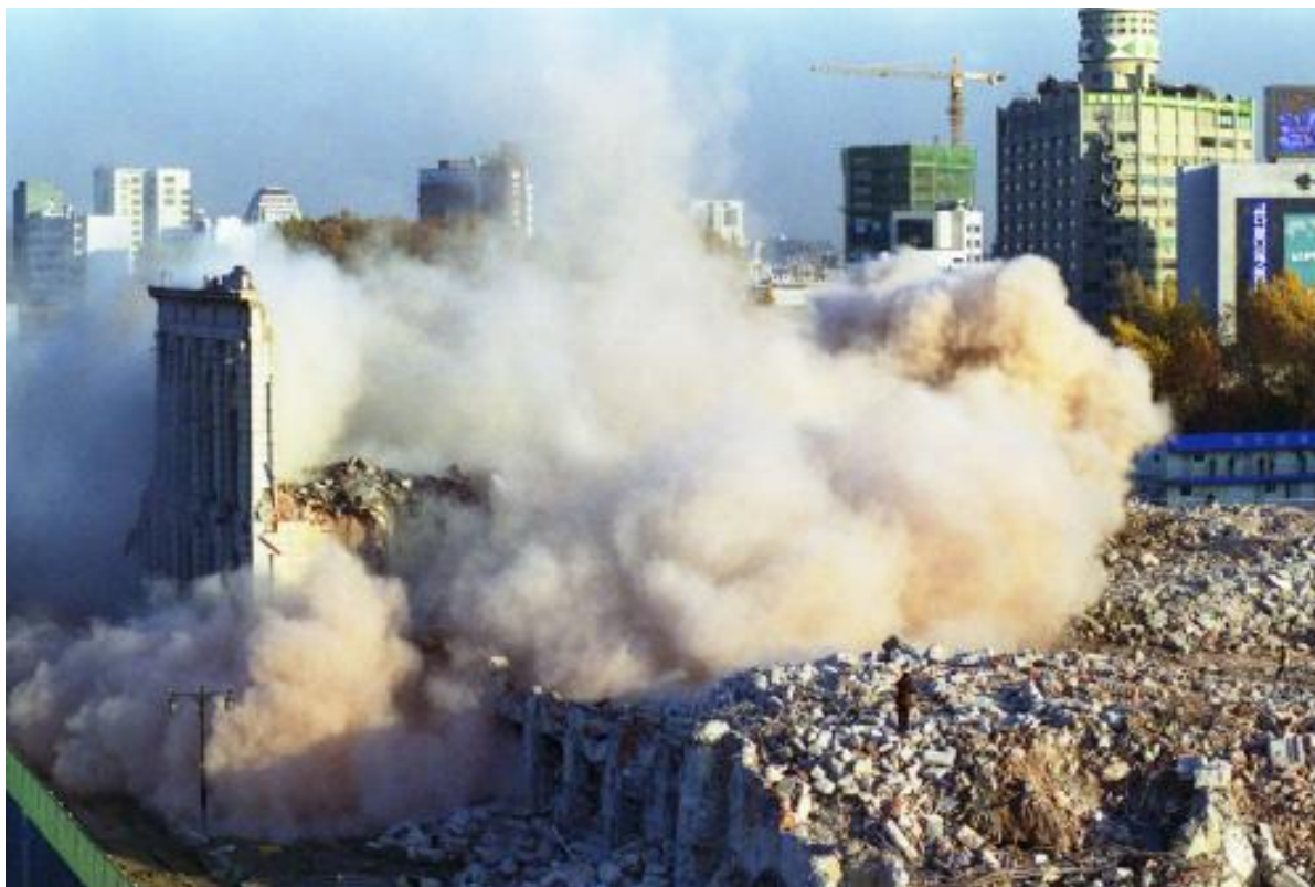
FIGURE 4-7. THE DEMOLITION OF THE JAPANESE GOVERNMENT-GENERAL OF KOREA BUILDING.
