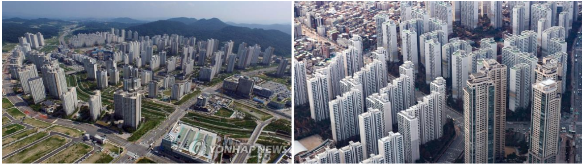
FIGURE 6-5. AERIAL VIEW OF A LARGE APARTMENT COMPLEX IN SEJONG (LEFT) AND SEOUL (RIGHT) SOURCE: (LEFT) HONG KUK-GI (2022); (RIGHT) YU YOUNG-GYU (2020).
