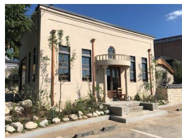
FIGURE 5-14. RESTORING MODERN HERITAGE IN GONJU. SOURCE: AUTHOR.
