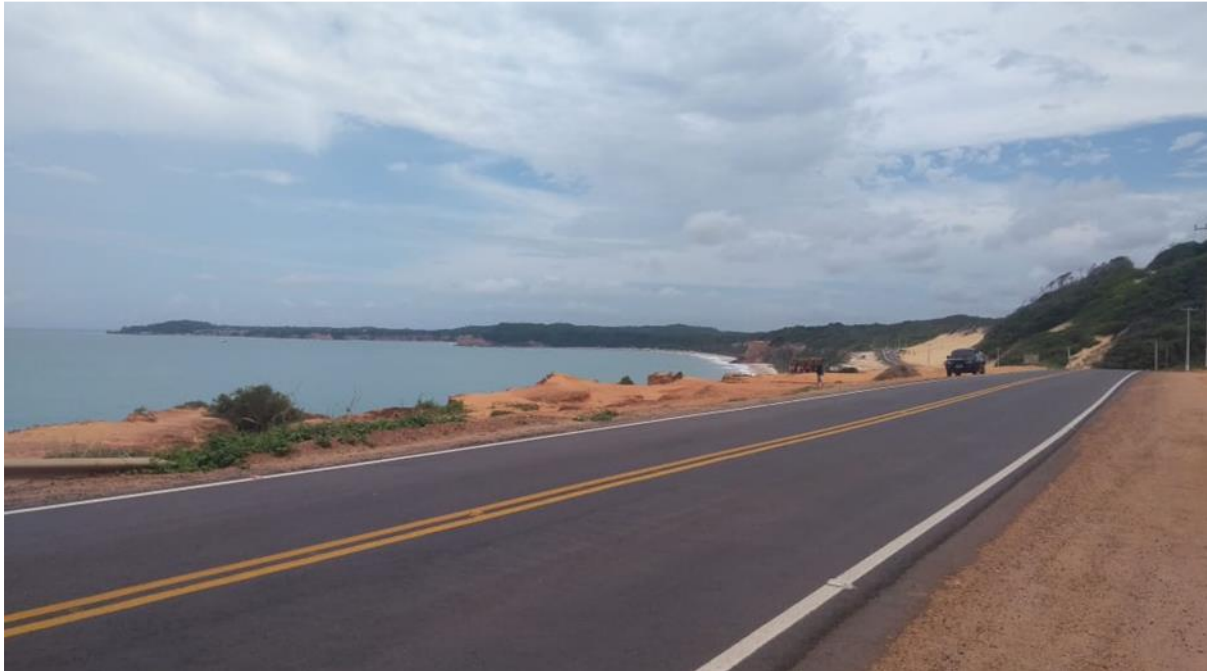
Figure 18 The new road surface on the approach to Pipa.
