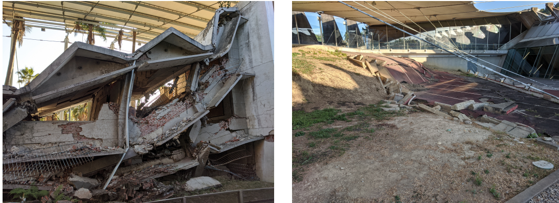
Figure 7.5: A school building damaged and the athletic field uplifted by 2 m in Kwang-Fu Junior High School.
