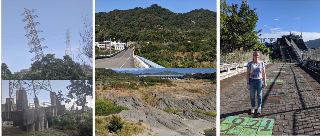
Figure 7.4: (left) Tilted tower moved by the event. (middle) Over the Dajia river, the Pifeng bridge got broken and the river bed got moved up of 6 m creating a waterfall (not visible anymore). (right) The northern end of the Shihgang dam truncated from the rest of the dam, the main part was uplifted by 9.8 m.
