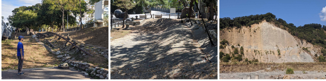
Figure 7.6: (left) Railway torned and uplifted. (middle) Parallel segment in the north showing 1 m uplift. (right) Fault scarp showing geological structures.
