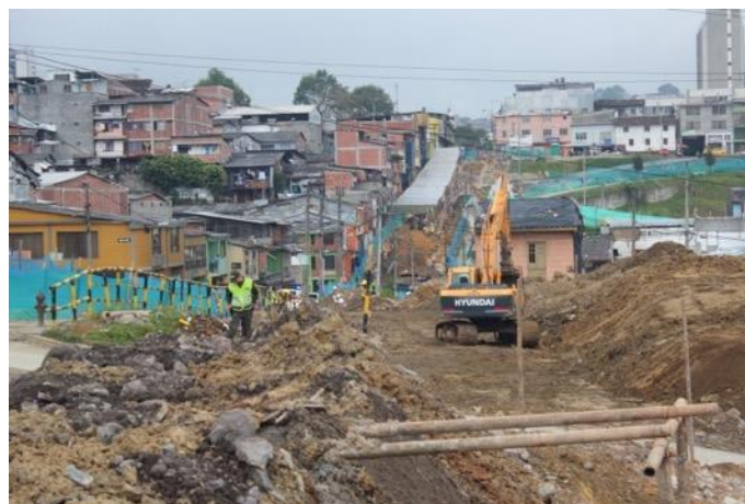
Image 15 Road works by the San Jose Macro-project. (Source: Caleidoscopios Urbanos (2016b))
