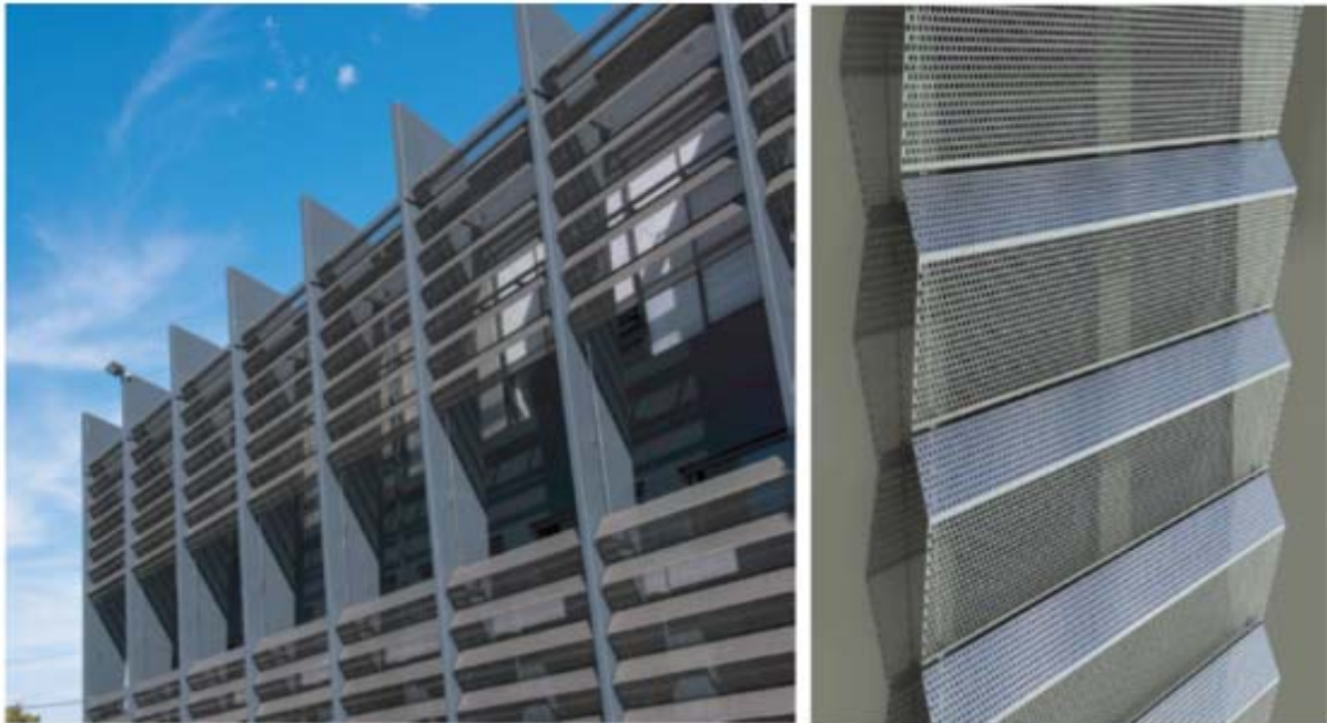
Figure 7.9: A systematic facade element which provides the occupants with maximum daylight and minimum solar radiation
