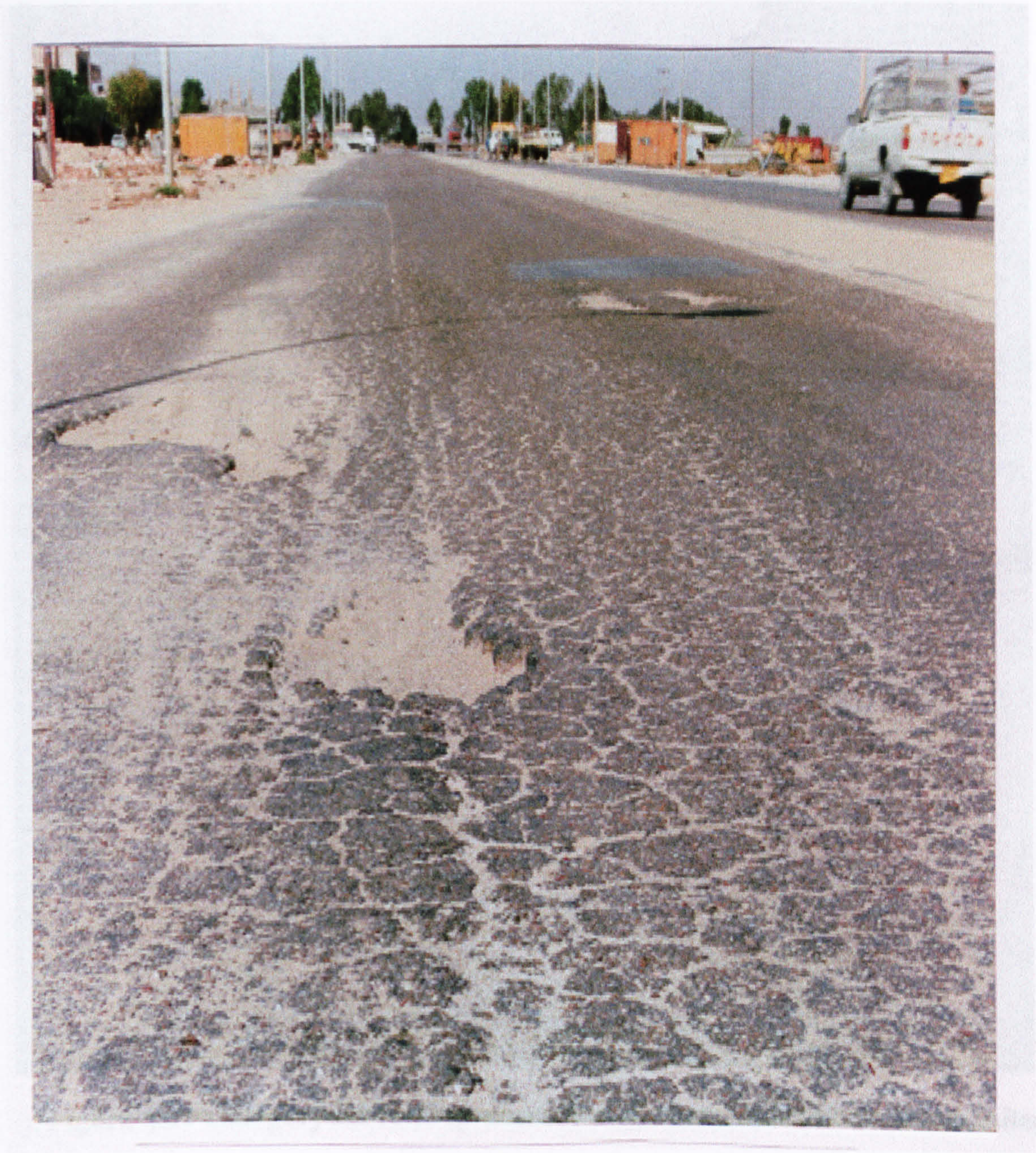
Figure 4.15 Category III road connecting 4 th and 5 th ring roads: Excessive cracks and potholes
