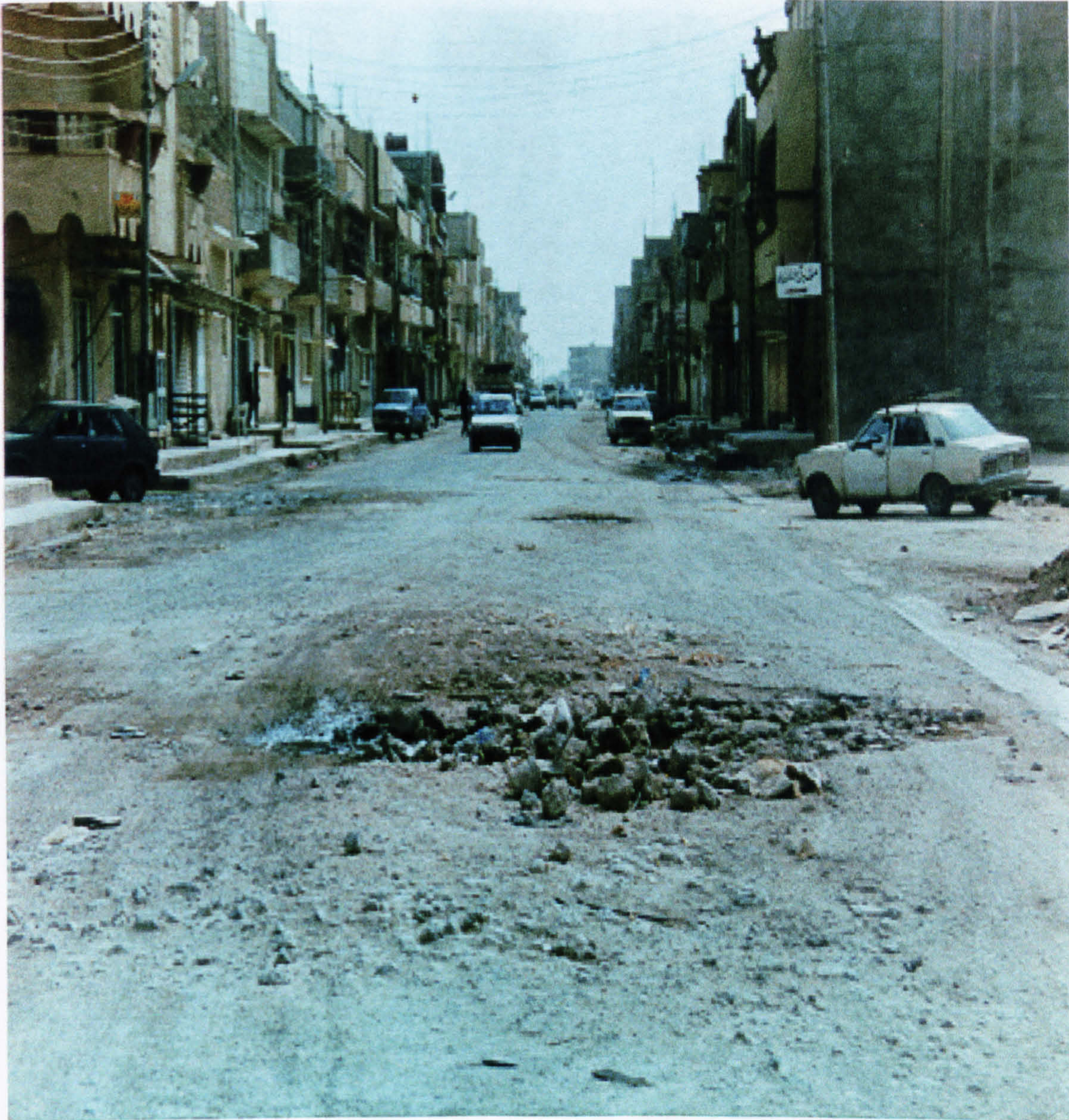
Figure 4.16 Category III road in unserviceable condition: Foundation failed
