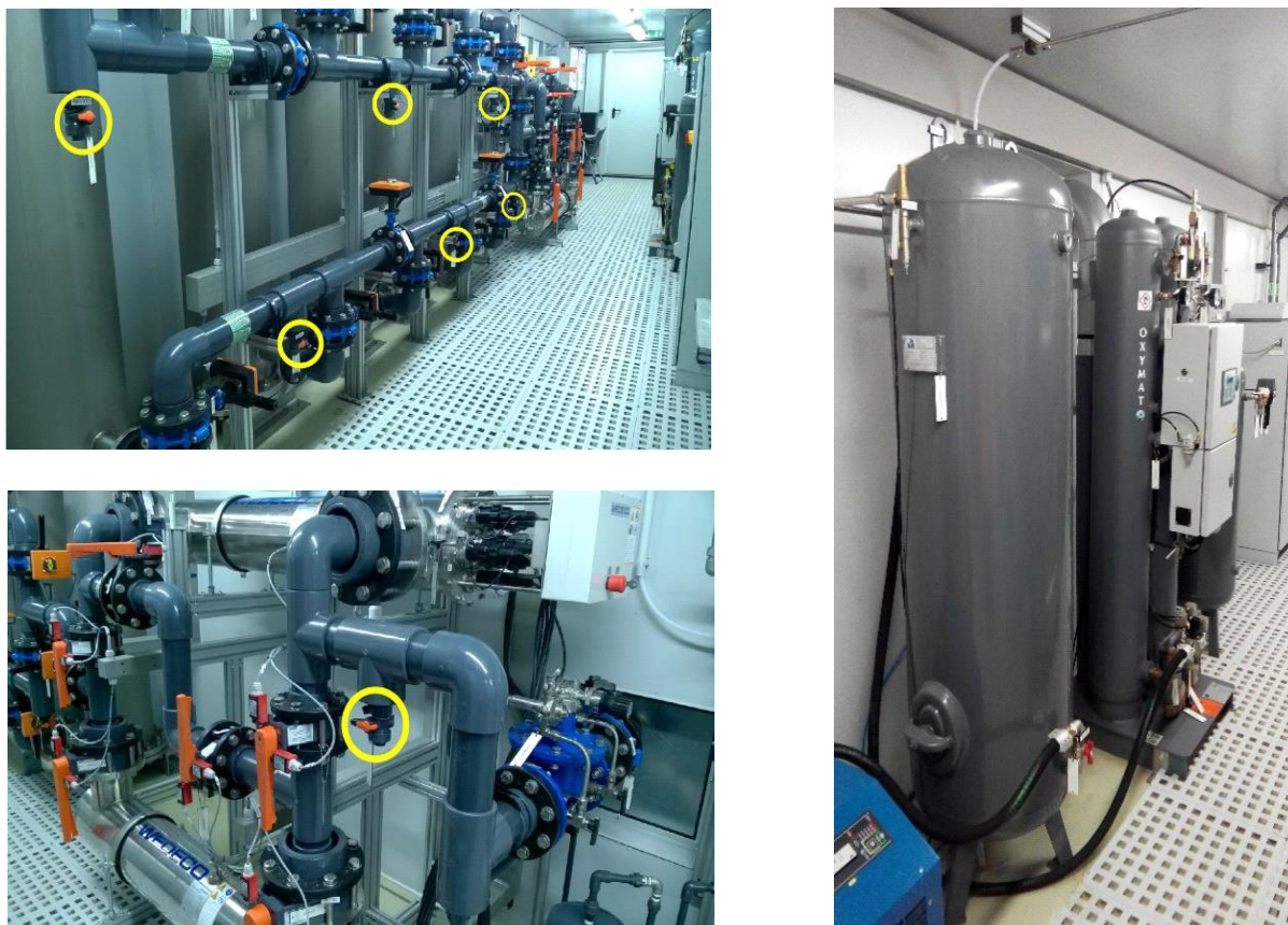
Figure 4.2 Sampling points highlighted upstream and downstream of the ozone and hydrogen peroxide contactors (left up) and UV system (left down). Ozone generator (right).
