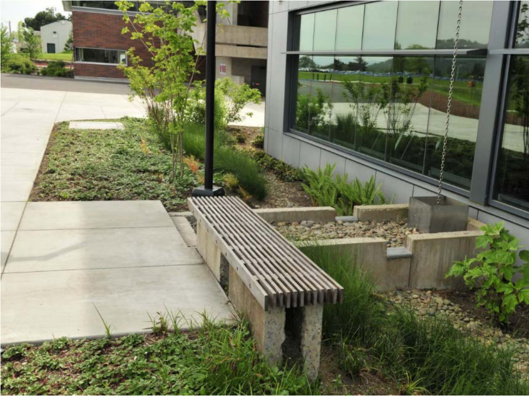
Figure 3: Example of shallow vegetated stormwater facilities integrated within site planting, Lane Community College Health and Wellness Centre, Eugene, OR
