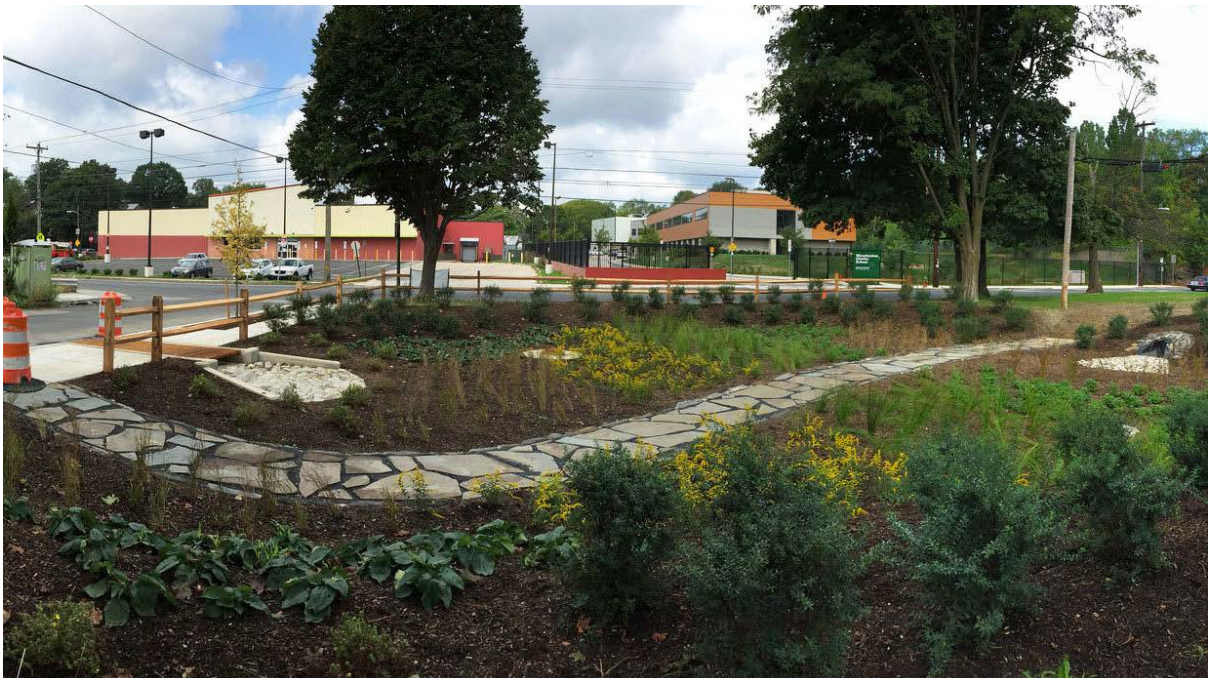
Figure 2: A rain garden manages stormwater runoff in Philadelphia's Germantown section (Philadelphia Water Department, unknown)
