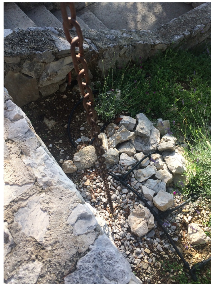
Figure 10: Rain chain and soak away, alongside irrigation pipes in Skradin. Croatia.
