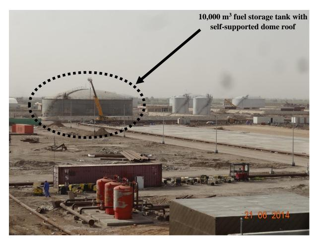
Figure 1.1 Site picture taken at Al-Samawa new depot project showing the general arrangement of the typical 10,000 m<sup>3</sup> storage tank investigated in this work.
