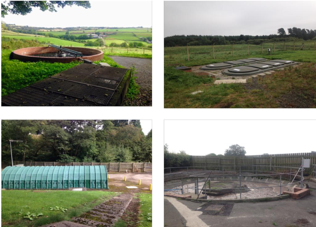
*Figure 1 - Examples of small WWTPs in NE England. Clockwise from top-left, technologies are trickling filter, high performance aerated filter, rotating biological contactor and activated sludge.*
