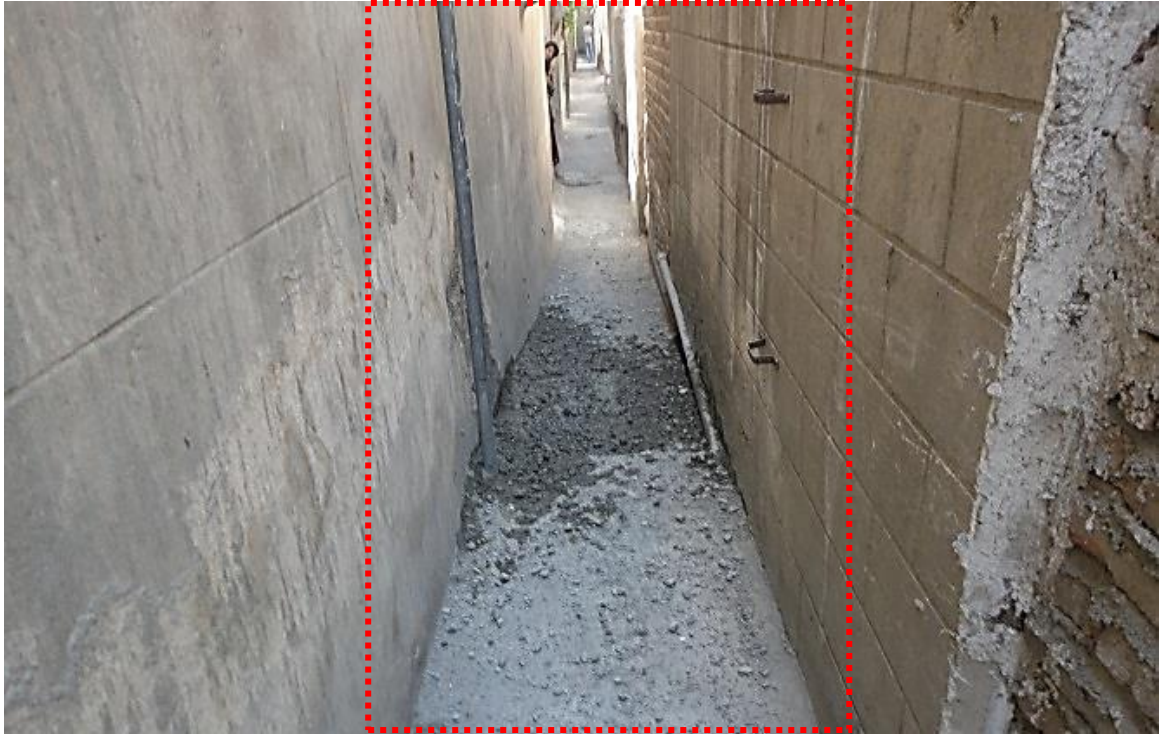
Figure 6.7 Materials spillage during construction (TM103-II)
