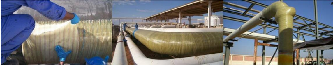
Figure 1.4: Pipe composite repair at Walker Technical Ltd.
