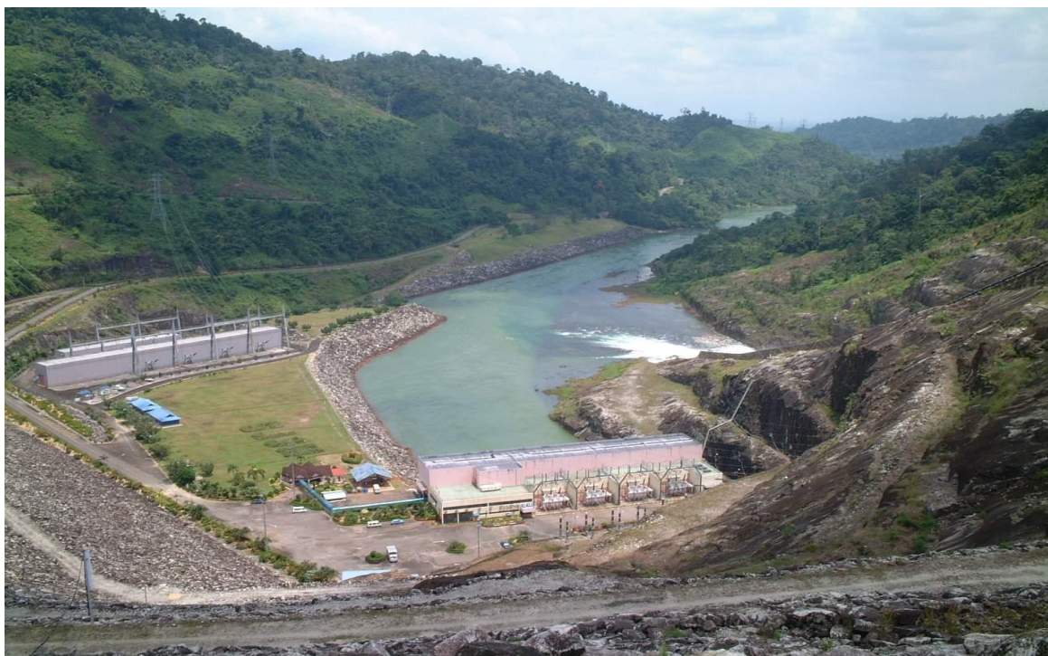
Figure 5.3: Sultan Mahmud Hydroelectric Power Station
