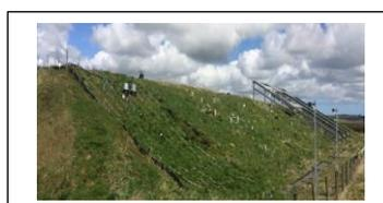
Fig. 2: The study site: instrumented embankment with distinctive well compacted and poorly compacted panels (b)
