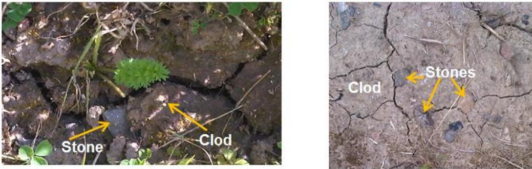
Figure 5.25: Polygonal cracks formed around stones and clods in exposed soil surfaces of the embankment
