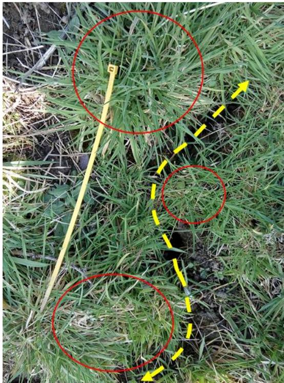
Figure 5.18: Vegetation influence on crack orientation in the embankment
