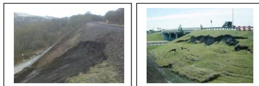
Fig. 1: The problem – slope failure like this can be activated by occurrence of cracks
