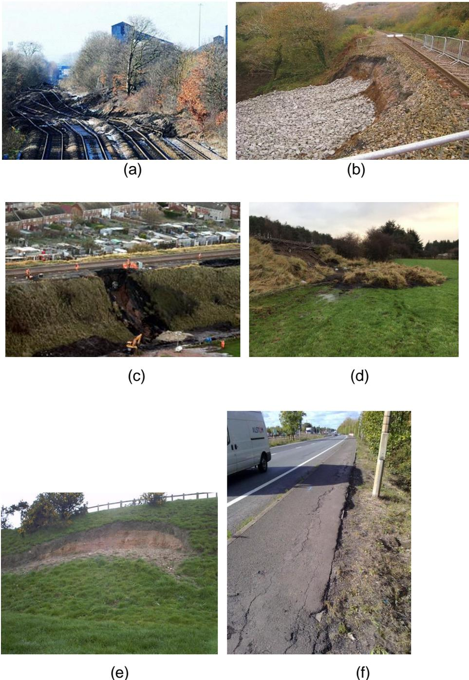
Figure 1.1: The problem: Different events and magnitude of earth slope failures affecting railways and highways transport corridor in the UK (photo a, b & c from ICE archives/Network rail; d & e from Briggs *et al.* (2016); from Electrokinetic Ltd, Newcastle University)
