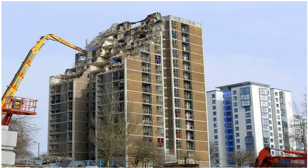
Figure Annex B1. ‘Last days of The Poplars’. Demolition of the Poplars building and the Hawthorns building (control building), recently refurbished, is to the right. Source: geograph.org.uk
