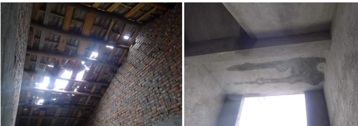
Figure 6.24 The damaged roof and floor of some new houses
