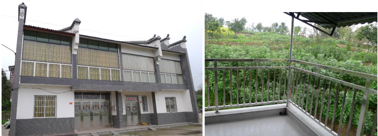
Figure 3.3 Photos of the glass curtain walls and the stainless steel components added on the house in Figure 3.2
