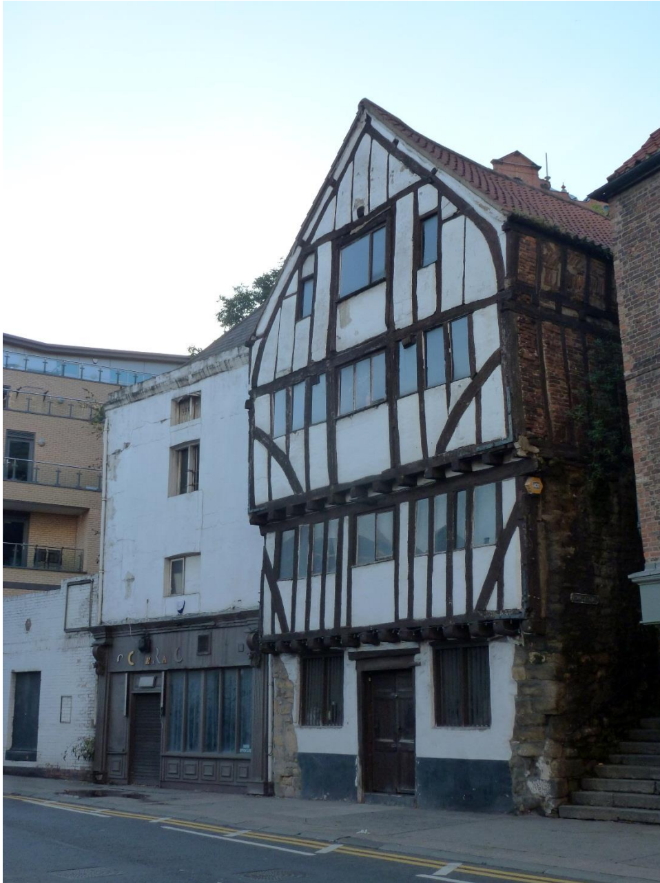
Fig. 7: The Cooperage, September 2016. Long Stairs and Merchant's Quay apartments are both visible. 13
