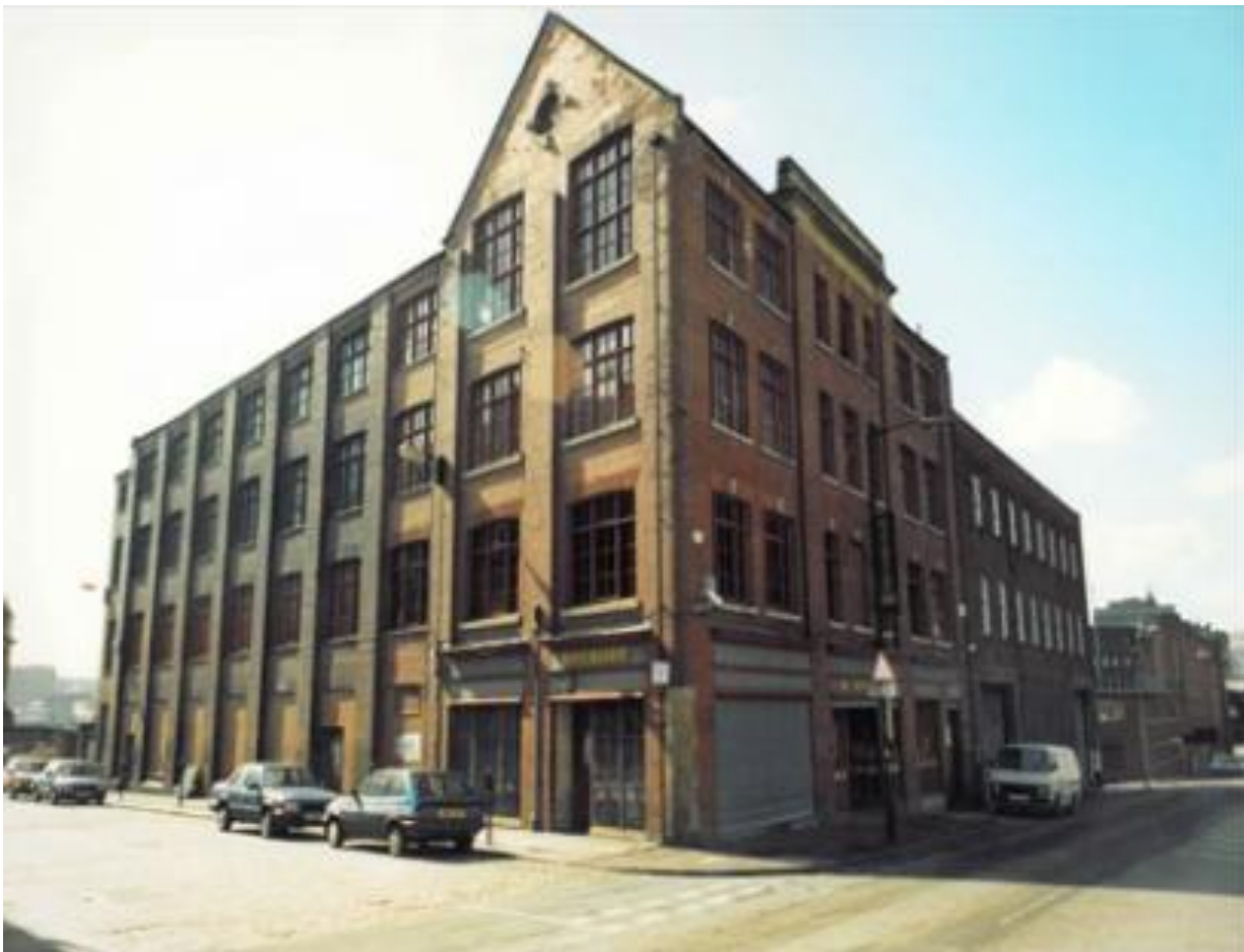
Fig. 6: Riverside, Melbourne Street, Newcastle. 2
