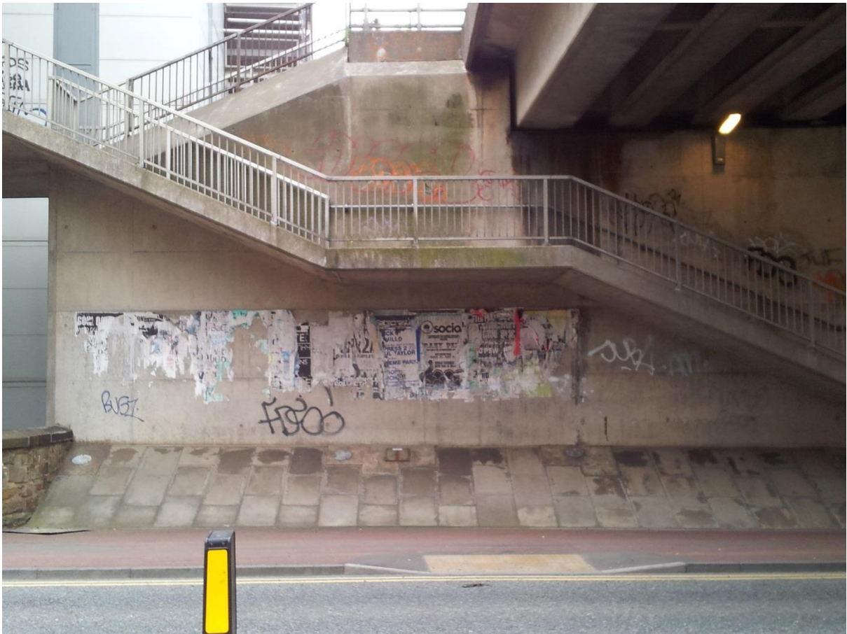
Fig. 11: Remains of old music posters beneath Redheugh Bridge, Newcastle, June 2016. 141
