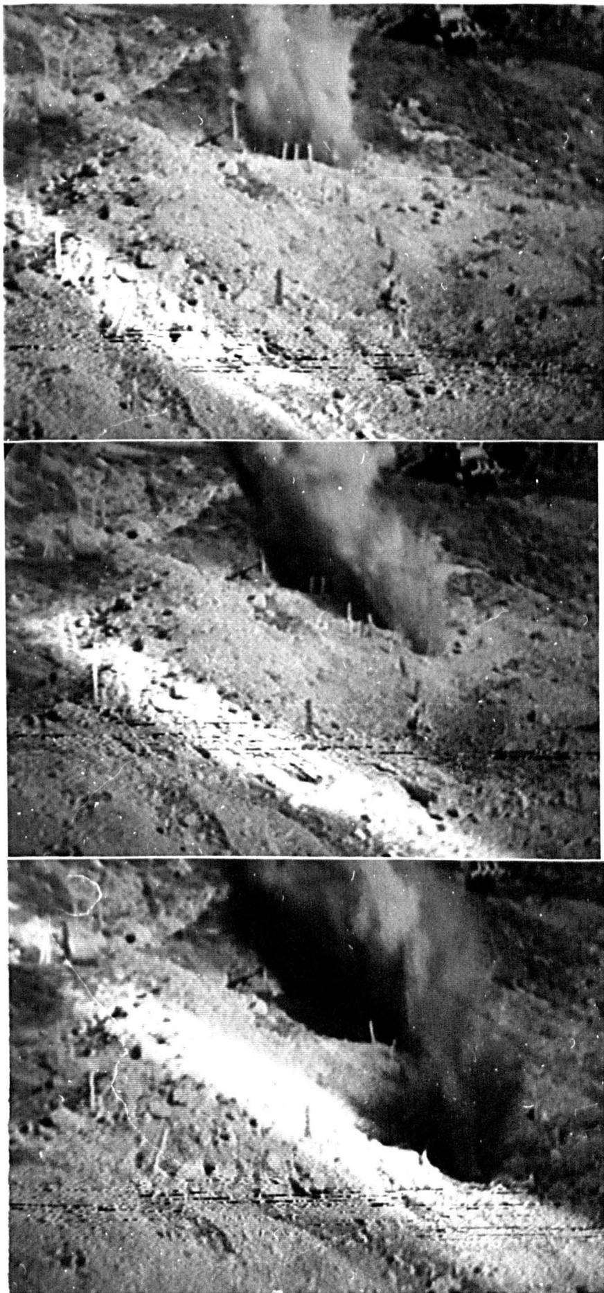
Fig.3.5. Video recording of pre-split panel at Location 9 showing sequence of detonation of 4 adjacent panels of 6 holes each (1-2-4-3).
