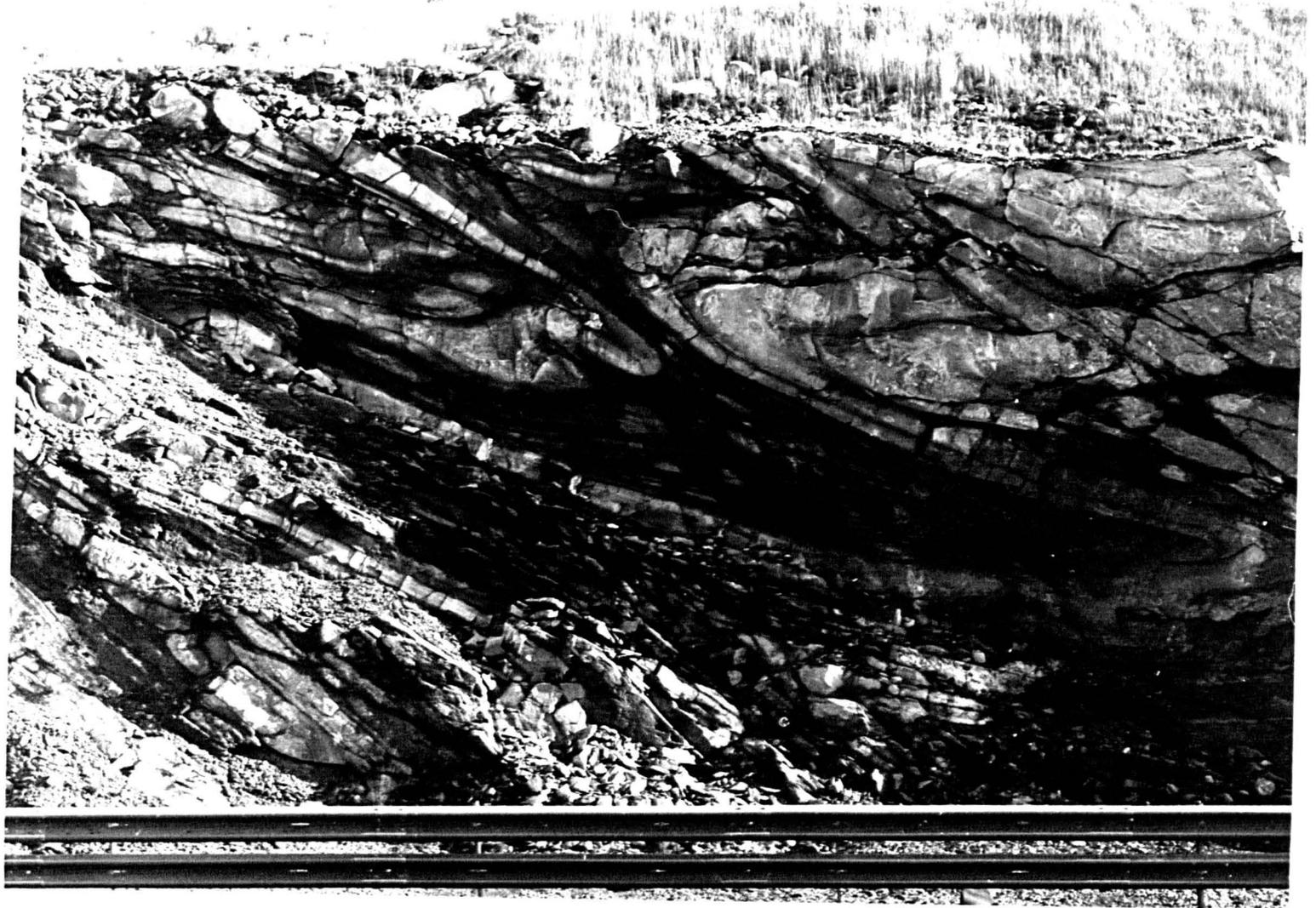
face with virtually no half barrels left visible in the resultant face. The final face is blocky in nature, reflecting the extent of continuity of the discontinuities and sits at a slightly lower angle of repose than designed.
