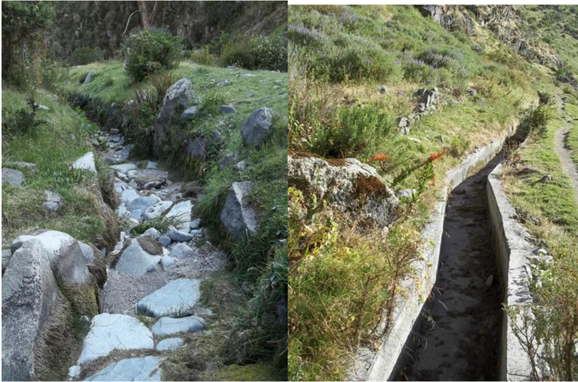
Figure 12 - (Left) The start of the Checa's Chaucalla canal, with 'alisados'. (Right) A newly refurbished section of Chaucalla canal close to the village nucleus in San Damián
