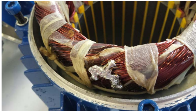
Figure 4.17 Stator interturn fault.
