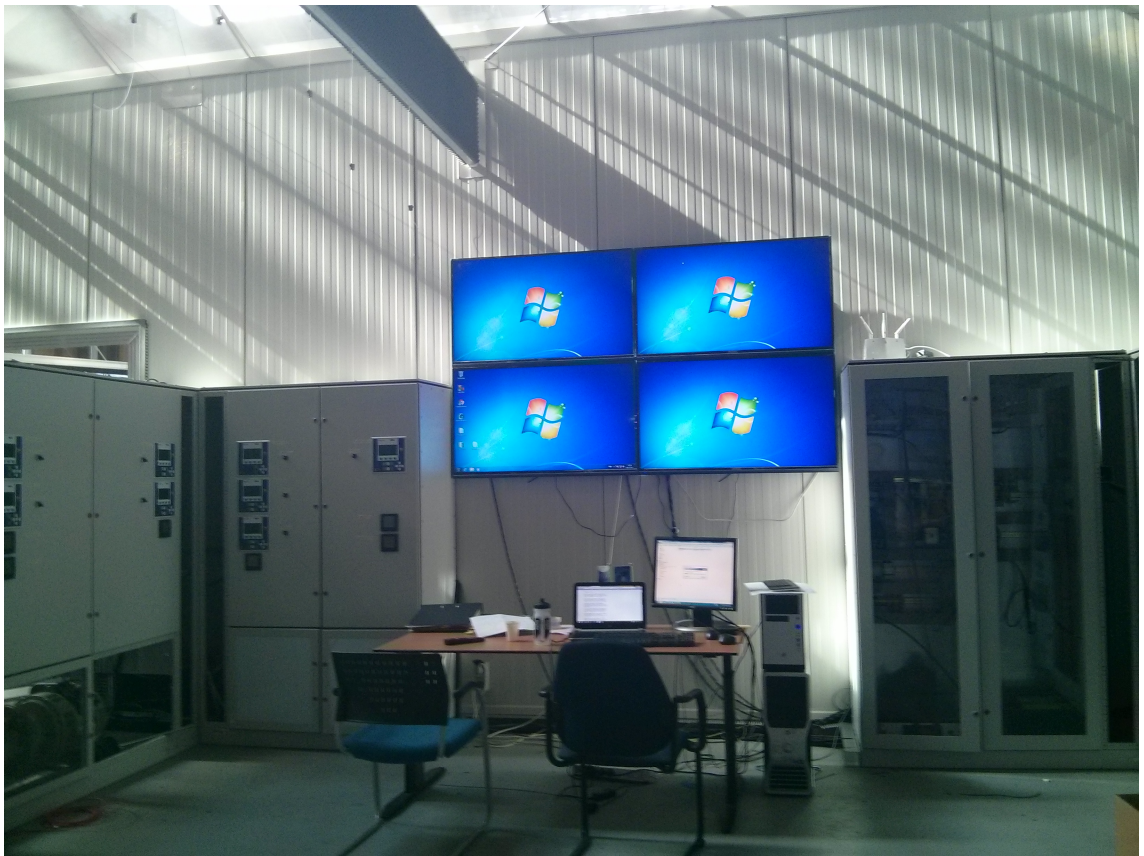
Figure 7.18 – Complete demonstrator view. HMI is displayed on the four central screens. EMS runs on the lower computer, while upper computer runs HMI system.
