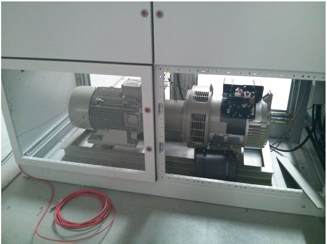
Figure 7.20 – Motor-generator pair emulating diesel generator.
