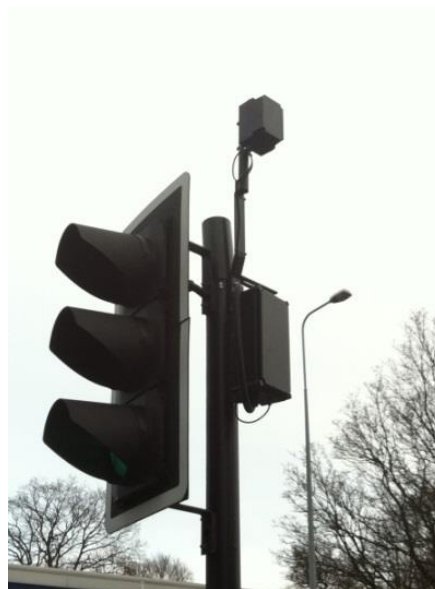
Figure 3.3: Typical Bluetooth Installed on a Traffic Signal Pole
