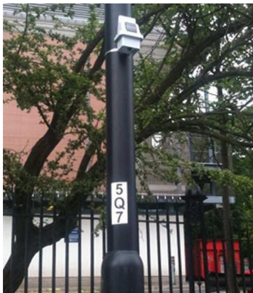
Figure 3.2: Typical Mote Installed on a Lamp Column
