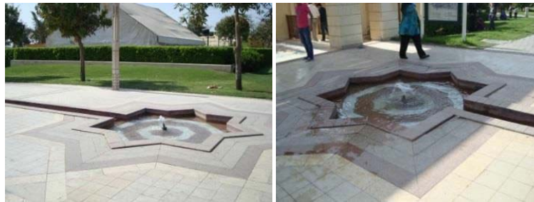
Figure 8.8: The two star-shaped fountains located at the beginning and the end of segment two
