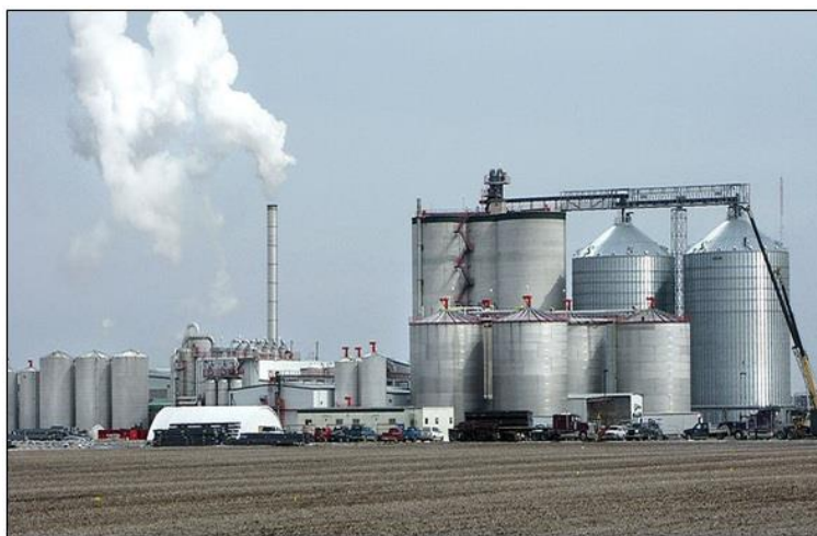
Figure 2.9: Ethanol plant in West Burlington, Iowa USA. ( www.wikipedia.org retrieved on the 14 February 2012).
