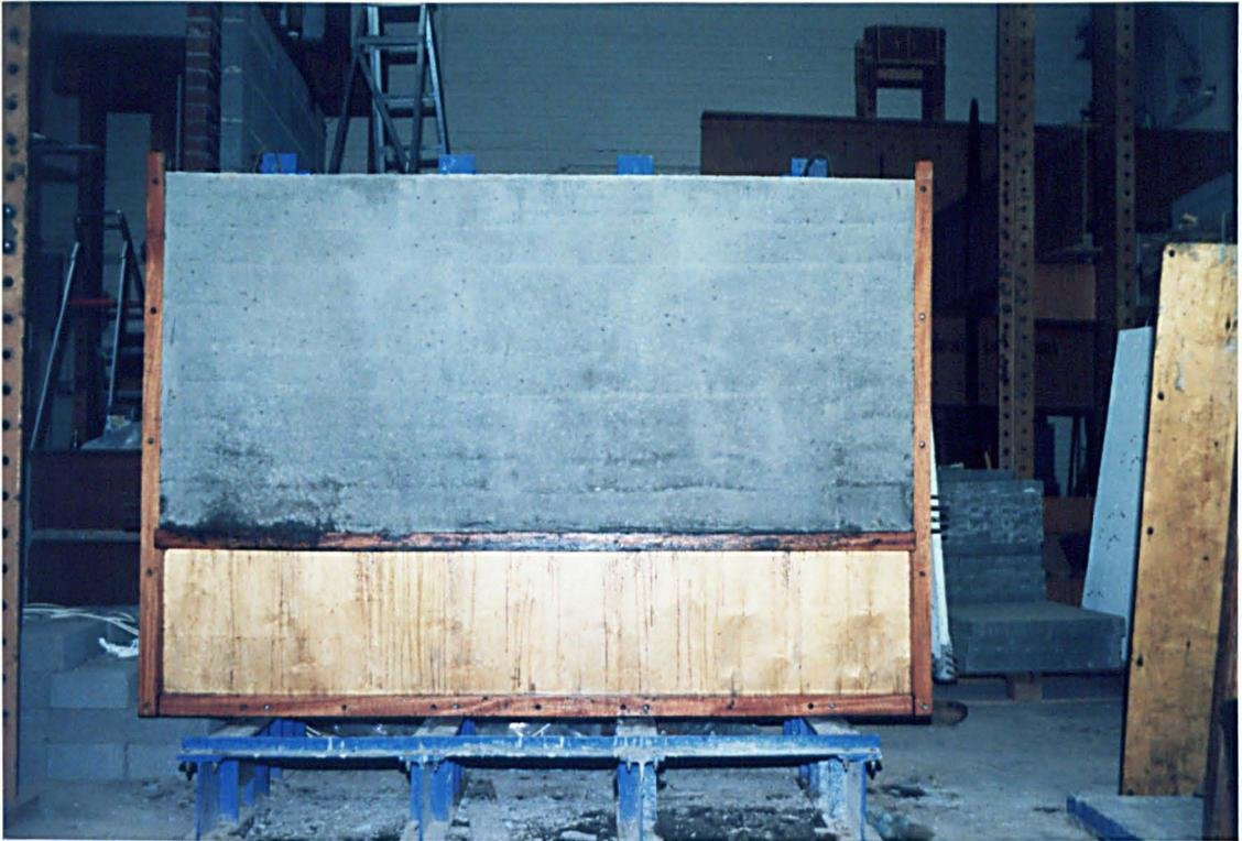
Fig.6.9: A beam being demolded from the big formwork
