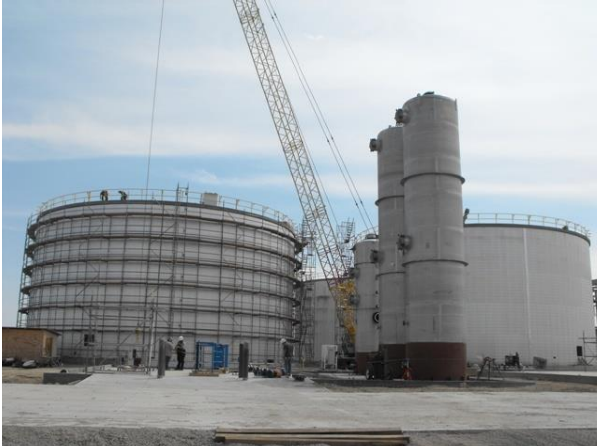
Figure 7.1 - Construction site works of an anaerobic digester at Kansas (ethanol plant with start-up planned soon); Dec. 2012 (Ethanol Produce Magazine, Dec. 2012).
