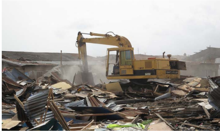
Figure 8.3: Demolition in Part of Badia Community Source: Channels Television (2013)
