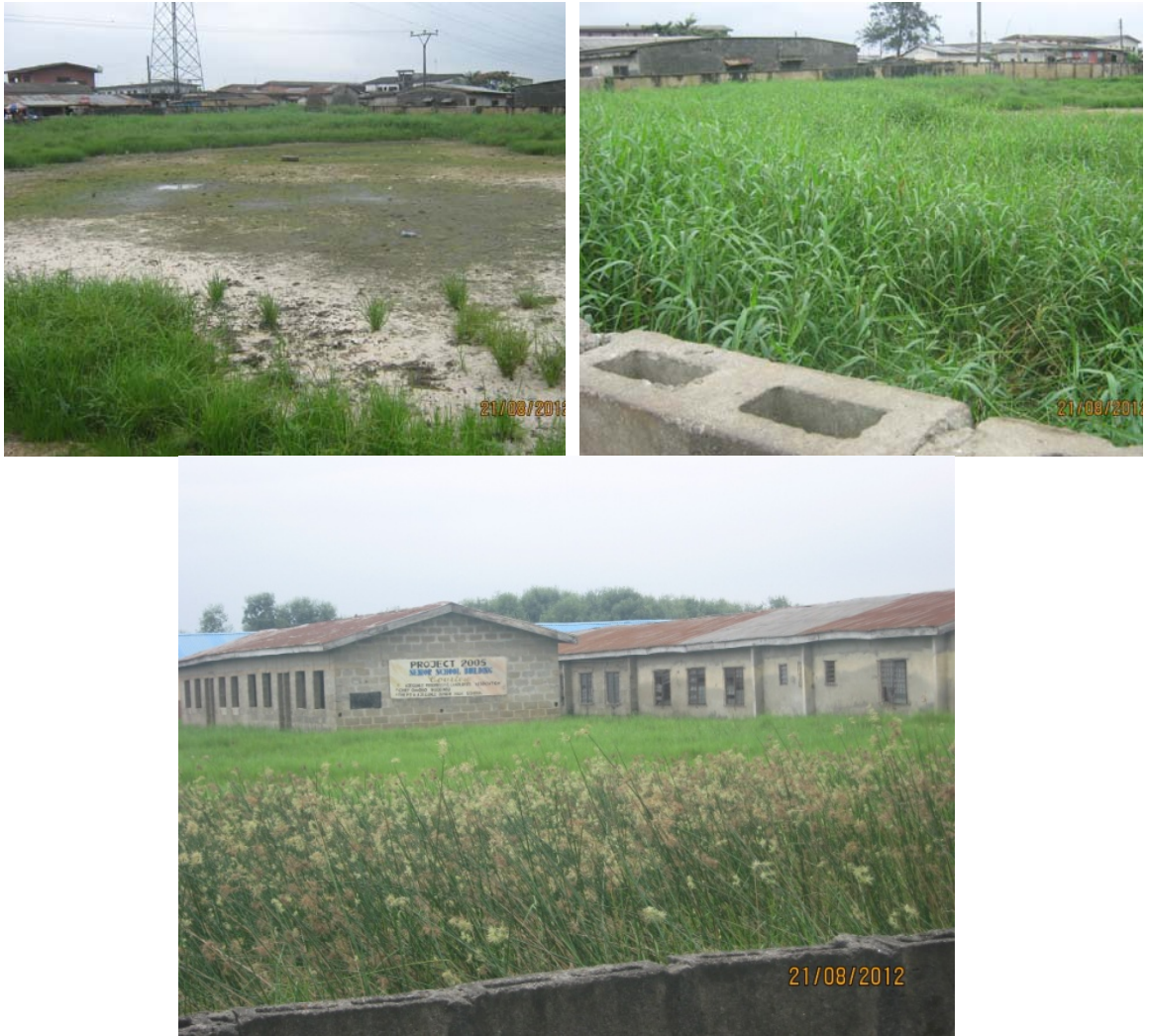
Figure 7.6: Ajegunle Secondary School Overgrown with Weeds as a Result of 2010 Floods.
