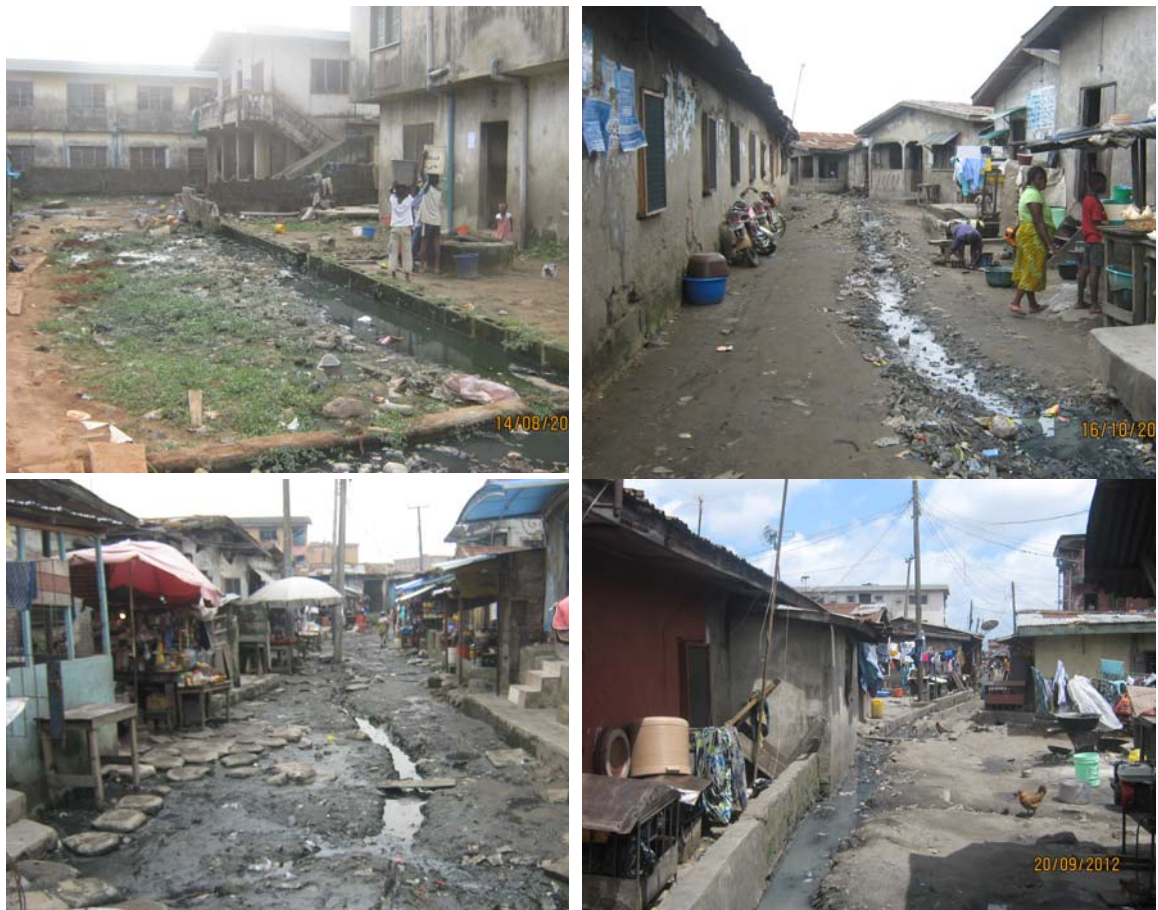
Figure 6.22: General Conditions of Access Roads and Drainage in the Study Settlements
