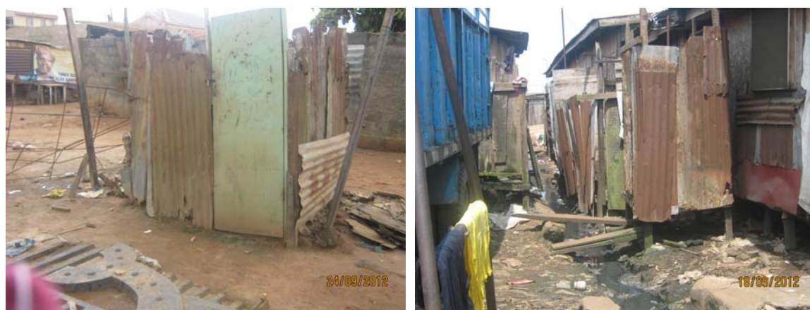
Figure 6.13: General Conditions of Toilets and Bathrooms in The Case Study Settlements
