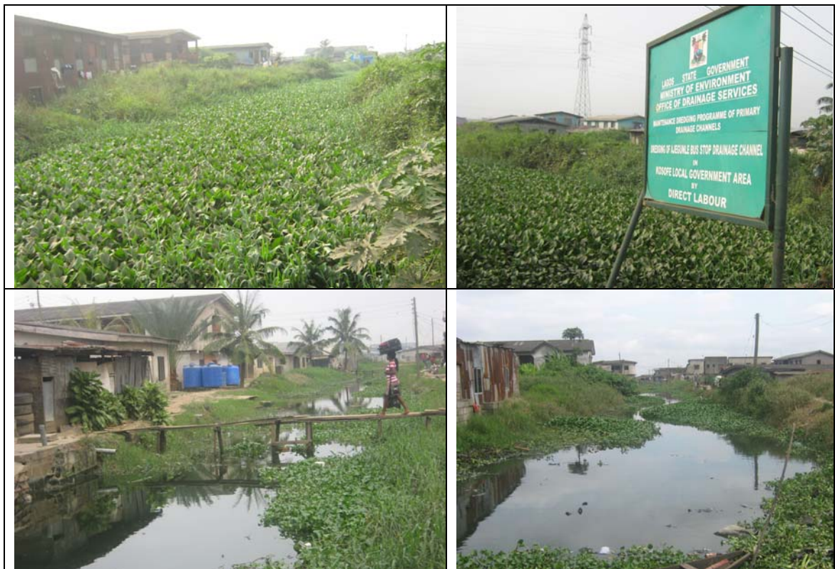
Figure 8.10: Abandoned Drainage Rehabilitation Work in Ajegunle
