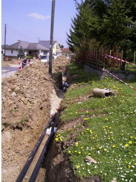
Figure 2. District heating system being installed at Güssing. Photo courtesy of Peter Vadasz
