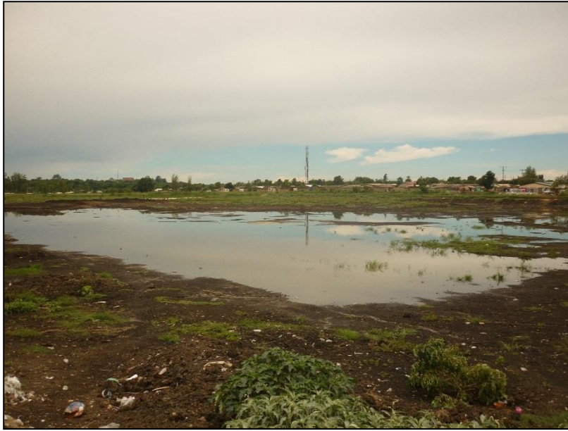
Figure 10-12: Stabilisation ponds following Manchinci WwTP
