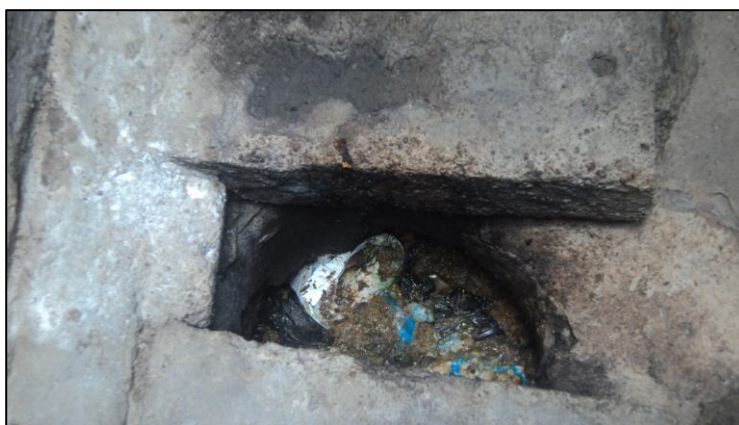
Figure 7-2 MSW observed in full pit latrine in Kanyama
