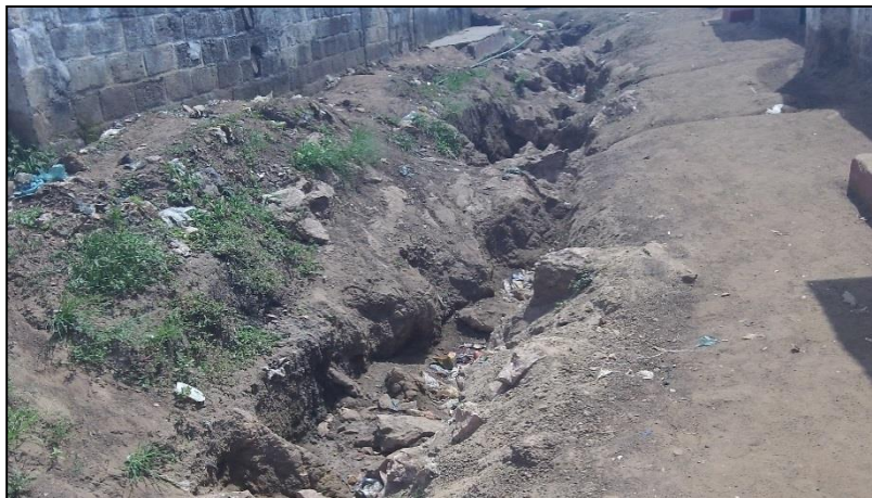
Figure 10-5: Drainage channel constructed in Kanyama
