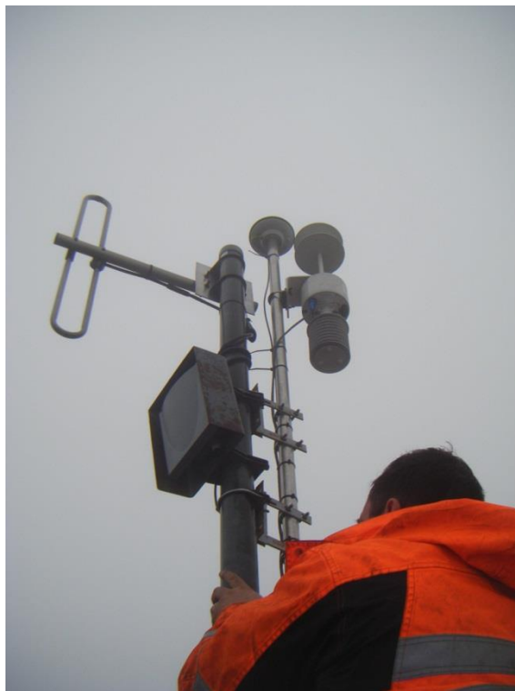
Figure 4-5. GNSS station on a stable platform (SNSU) with Leica AS10 GNSS antenna and co-located Met4 sensor.
