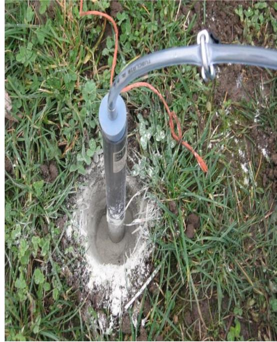
a) Careful installation into augered hole    b) Backfilling to create hydrological isolation
