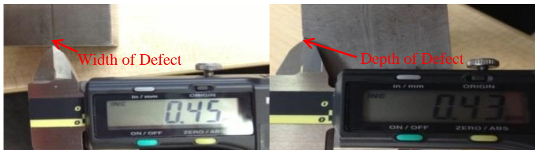
Figure 5.15 One small defect under measurement.
