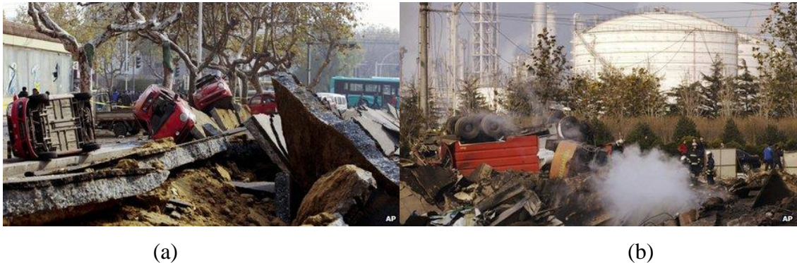
Figure 1.1 (a) The 2013 pipeline explosion in Qingdao damaged cars and the road in Shandong province. (b) 55 people were killed after the explosion [4].
