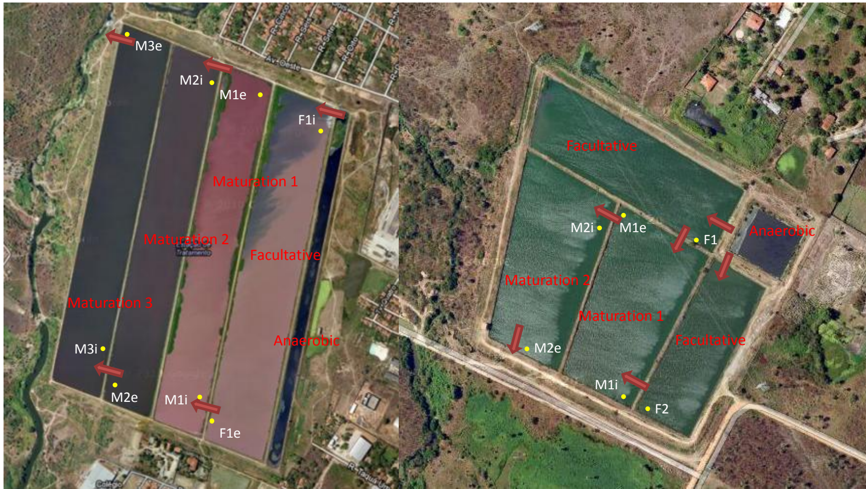
Figure 7-1 Satellite images (Google Maps) of the two WSP systems, SIDI on the left and Marechal Randon on the right. Arrows show the location of the inlet and outlet pipes, yellow dots and writing in white shows the sample collection points and names. SIDI is located at 3°51'19" S, 38°37'24" W and Marechal Randon at 3°46'44" S, 38°38'11" W.
