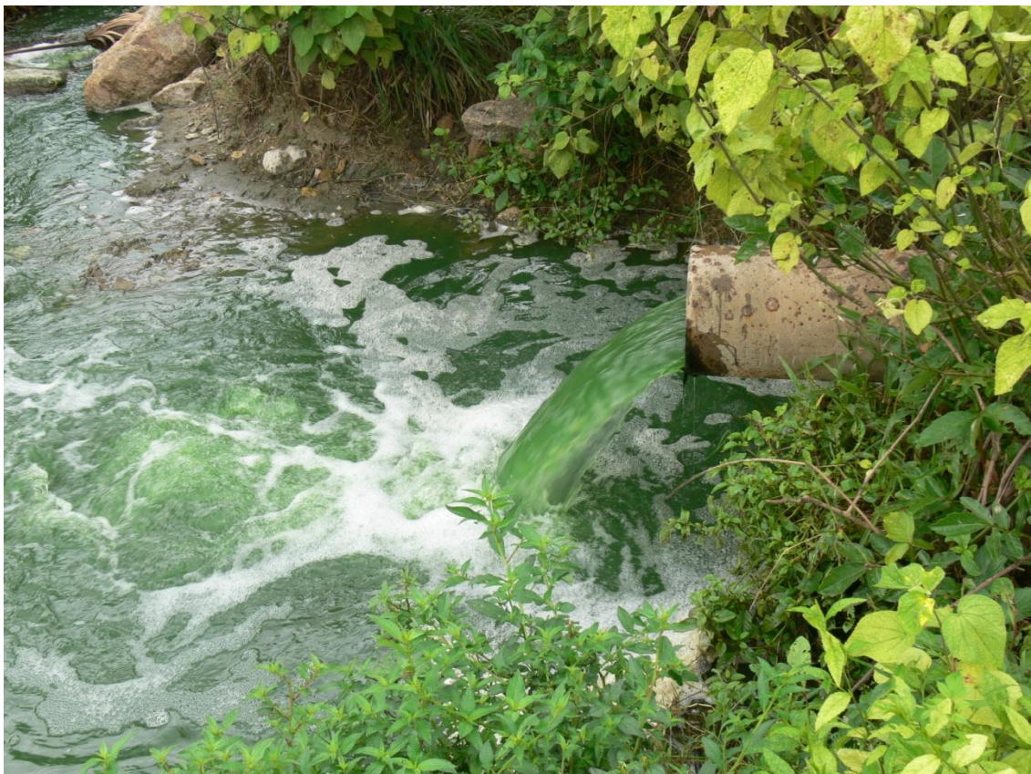
Figure 1-3 A photograph of effluent containing algal biomass leaving the Marechal Randon WSP system in Ceará, Brazil. (Photograph taken by Lucy Eland)
