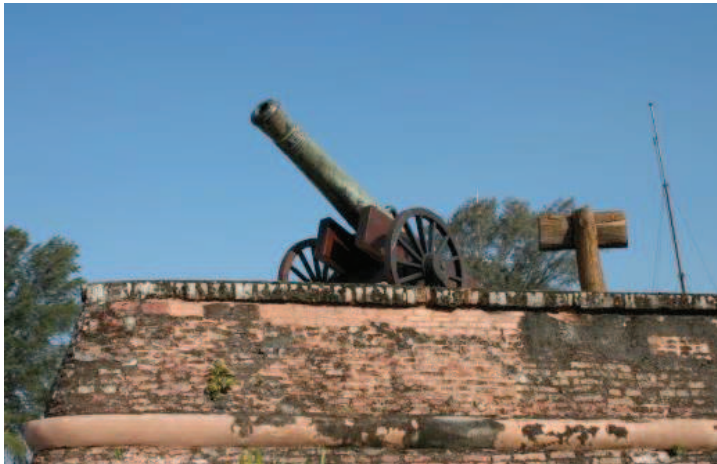
Photo 6.3: Site 3 - Fort Cornwallis
