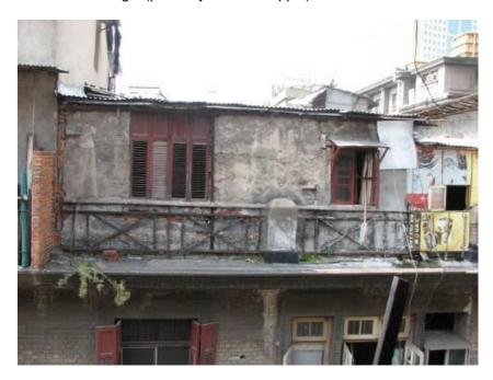
Figure 51 A rooftop extension sanctioned by the official authorities, distinguishable by its tiled roof (photo by Graham Tipple)
