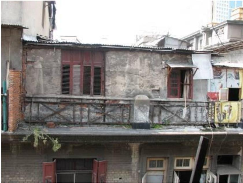
Figure 51 A rooftop extension sanctioned by the official authorities, distinguishable by its tiled roof (photo by Graham Tipple)
