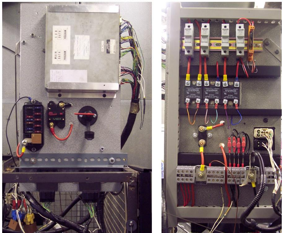
Figure 4.5: ECU and power distribution plate front (left) and rear (right)
