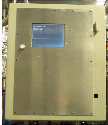
Figure 4.6: Dynamometer power electronics and control box in new engine cell
