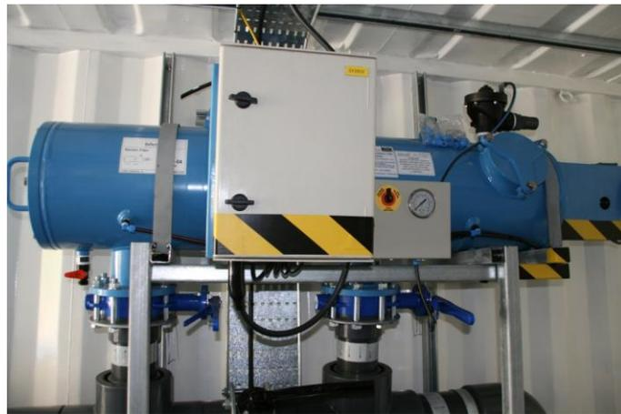
**Figure 4-5: Micro-filter with 40 micron screen**
