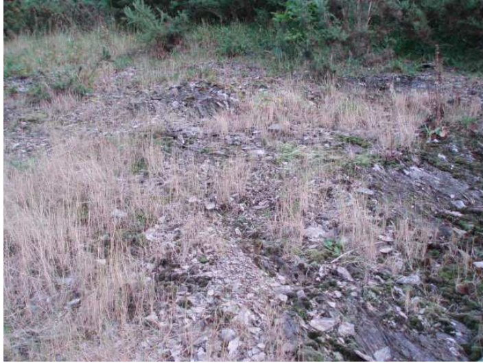
Photo 5.4. A38. South-facing bareground, signs of surface erosion on slate.
