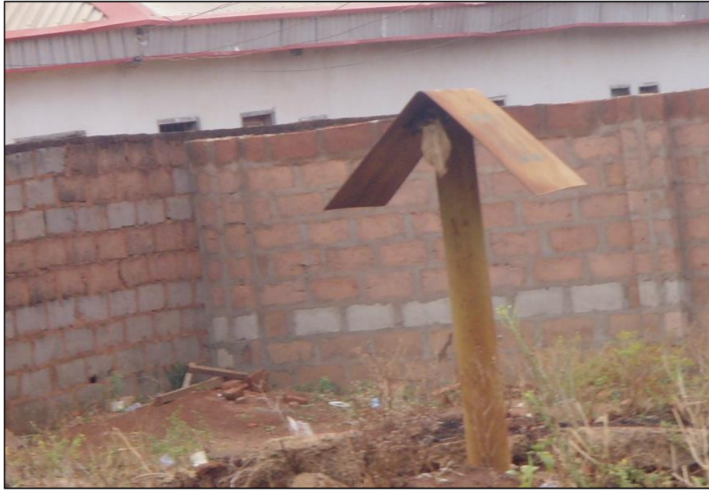
Figure 9: A dwelling unit encroaching on a pipeline
