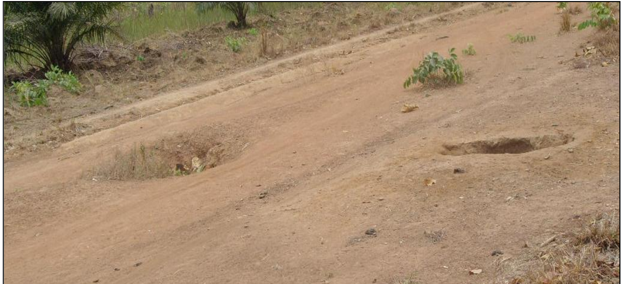
Figure 37: Holes made by vandals in search of pipeline in Otukpo
