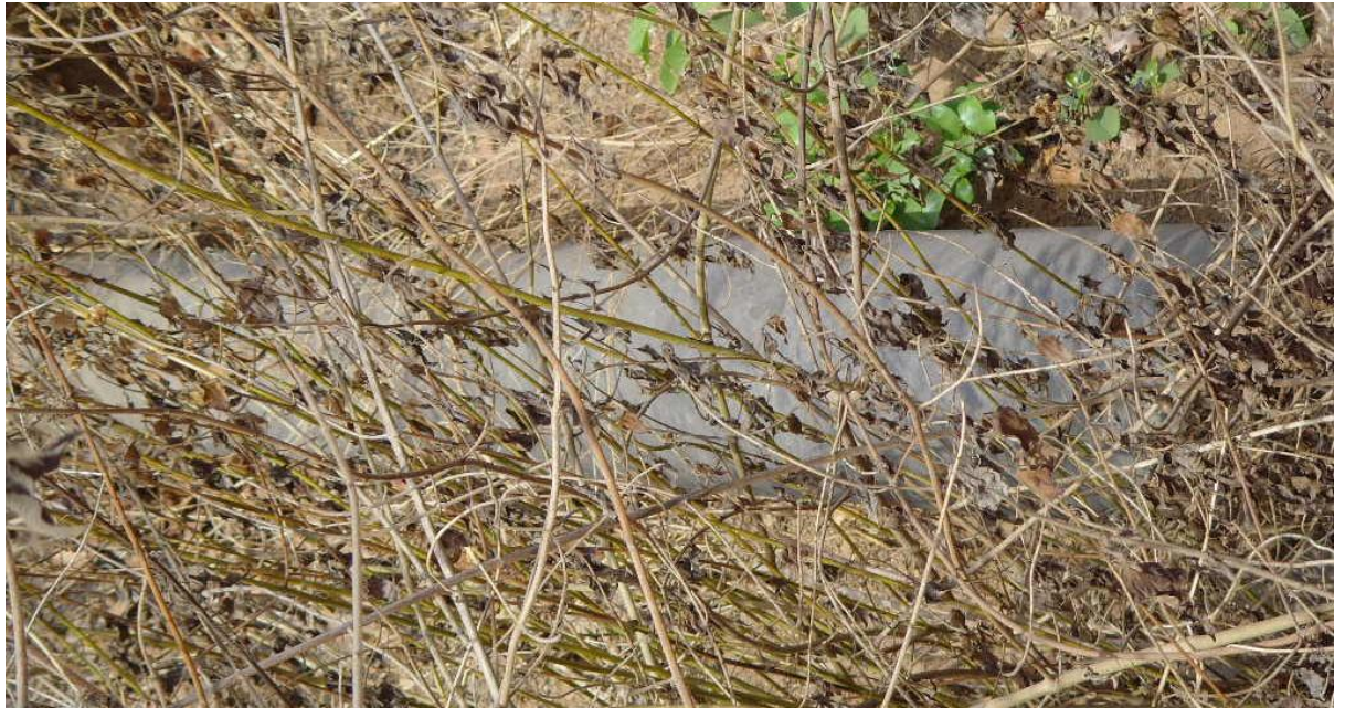
Figure 8: Showing a stretch of oil pipeline covered by vegetation
