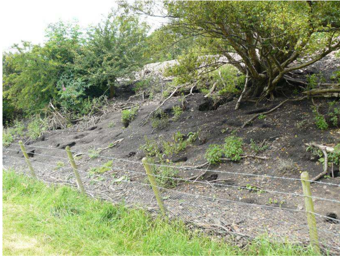
Figure 3.5 Part of a cutting earthwork approximately 2.5 km east of Haltwhistle. Here, tall shrubs dominate as well as large areas of bare earth. Much of this earthwork is riddled with rabbit holes presenting an additional problem to the network operator. Note the leaning fence posts indicating slope movement.
