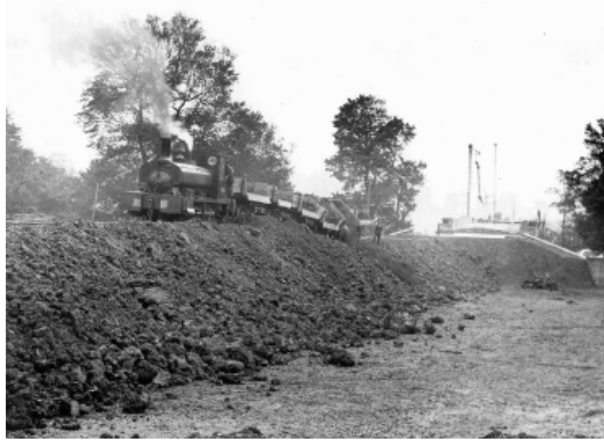
Figure 1.1 Embankment construction in 1922 using a steam powered locomotive to tip material on the earthwork from Perry et al. (2003b).
