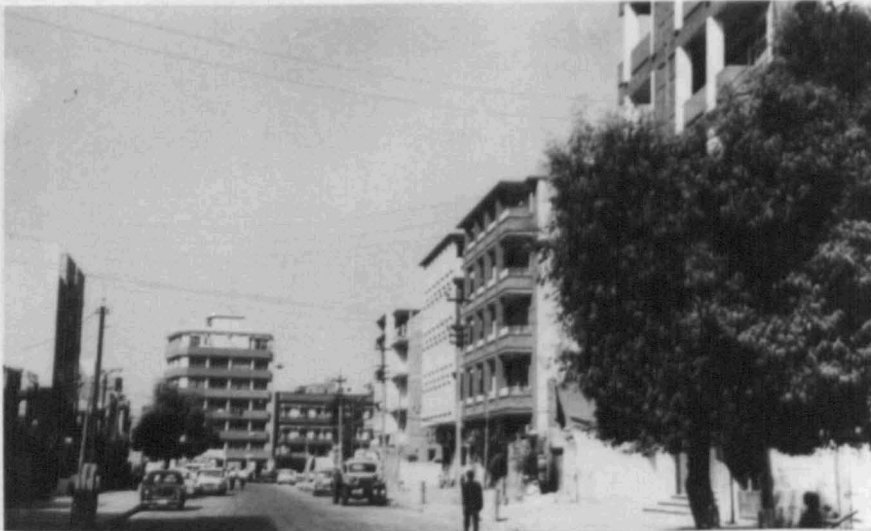
b. Al-Sadun and its tributary side streets are undergoing functional and thus morphological change
