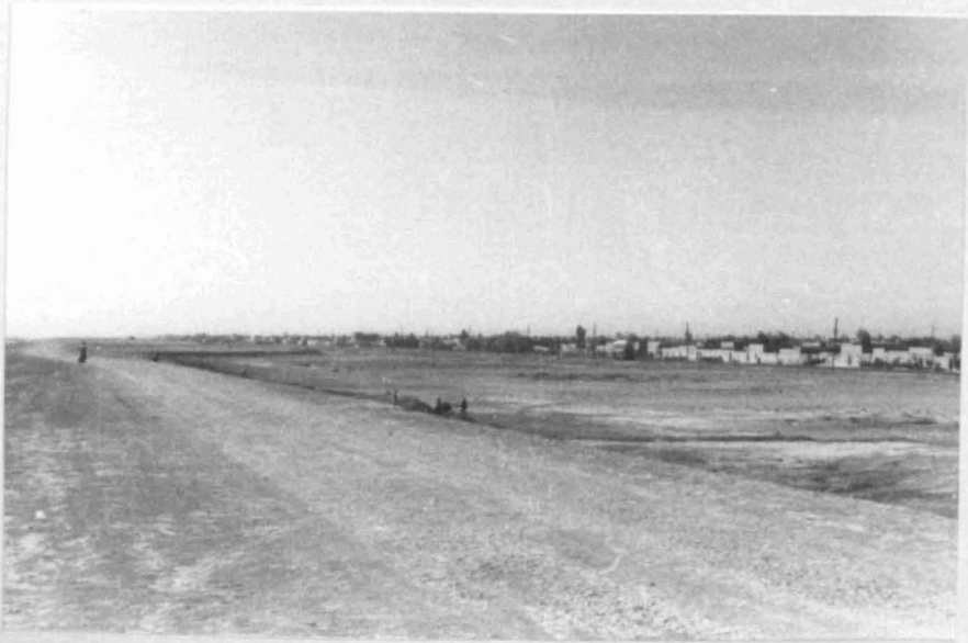
b. The new dyke, al-Saddah al-Shamaliyah, surrounding most of the modern development of the East Side for flood control
